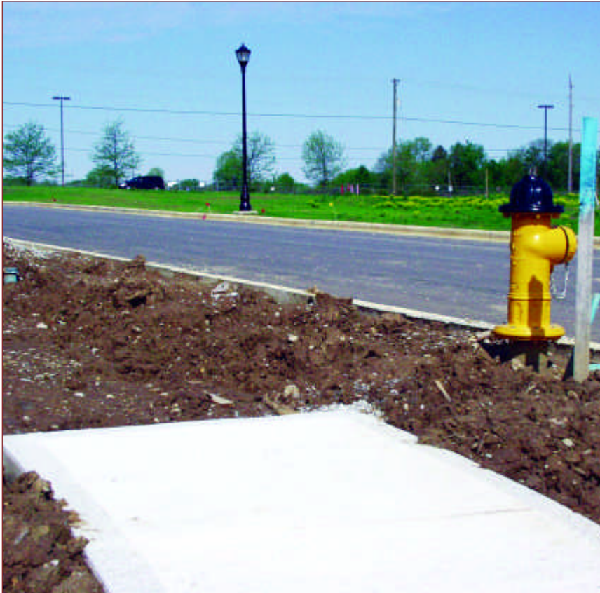
New sidewalks, streetlights and utilities in Alum Creek Village.
