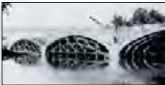
North Broadway Bridge construction. (Source: Franklin County Engineers)
