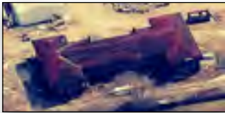
Laneview School on Kenny shortly before it was demolished. (Source: Google Earth)
