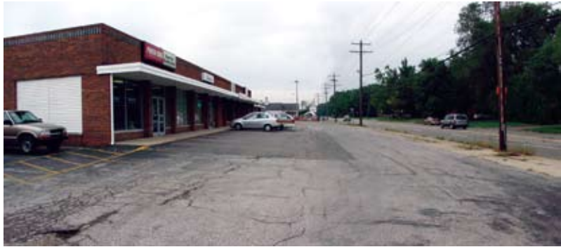
Indianola Avenue at Wetmore Road- Before
