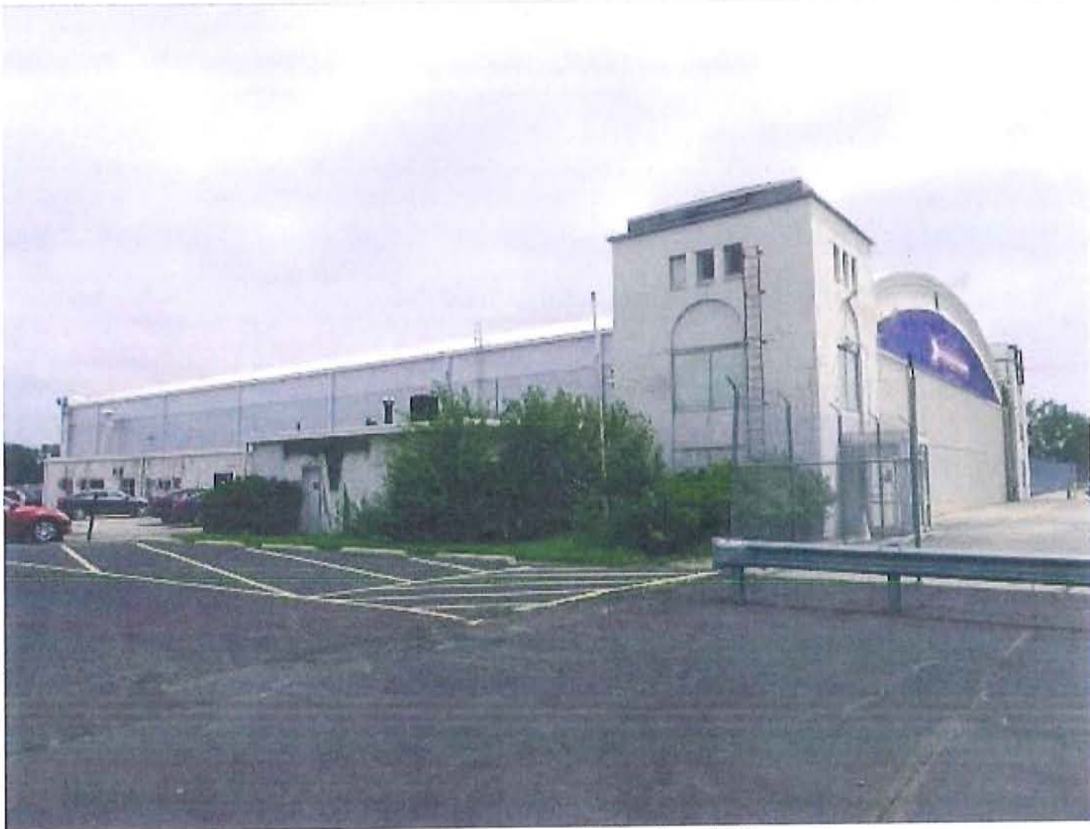
15. TAT Hanger, west and north elevations, looking southeast
