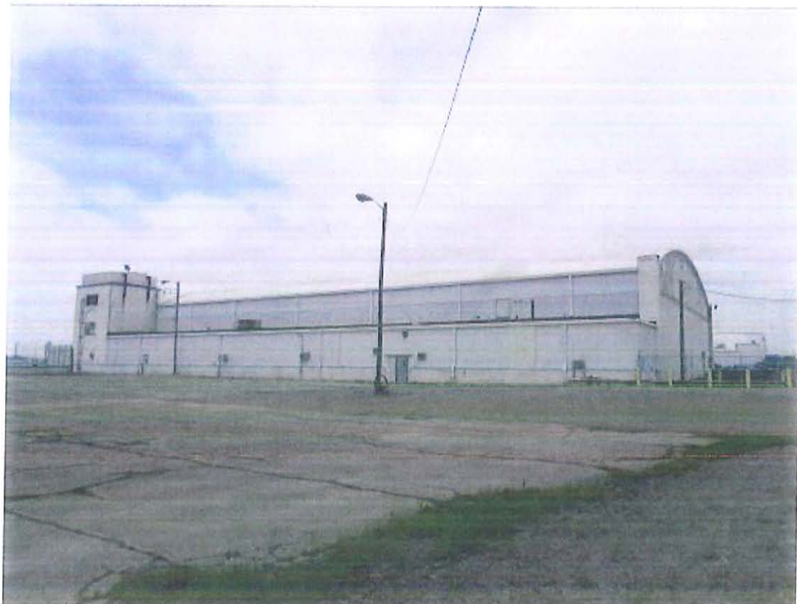
14. TAT Hanger, south and east elevations, looking northwest
