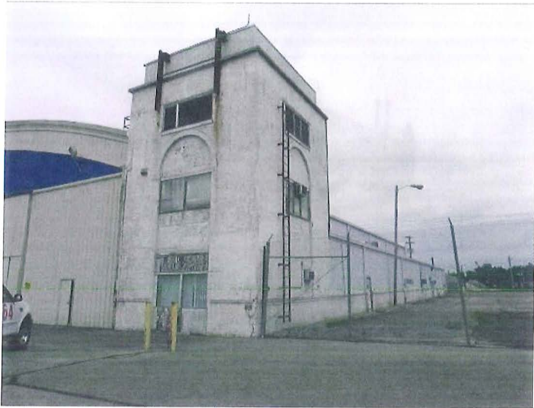
13. TAT Hanger, west and south elevations, looking east
