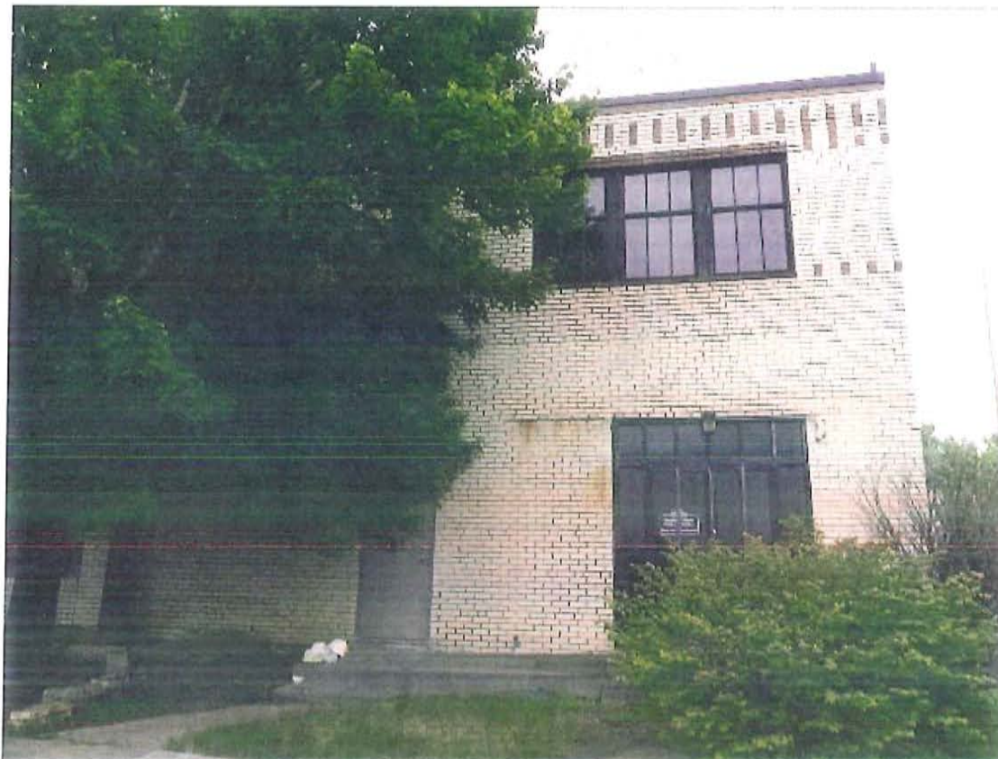
6. Passenger Terminal, west elevation, looking east
