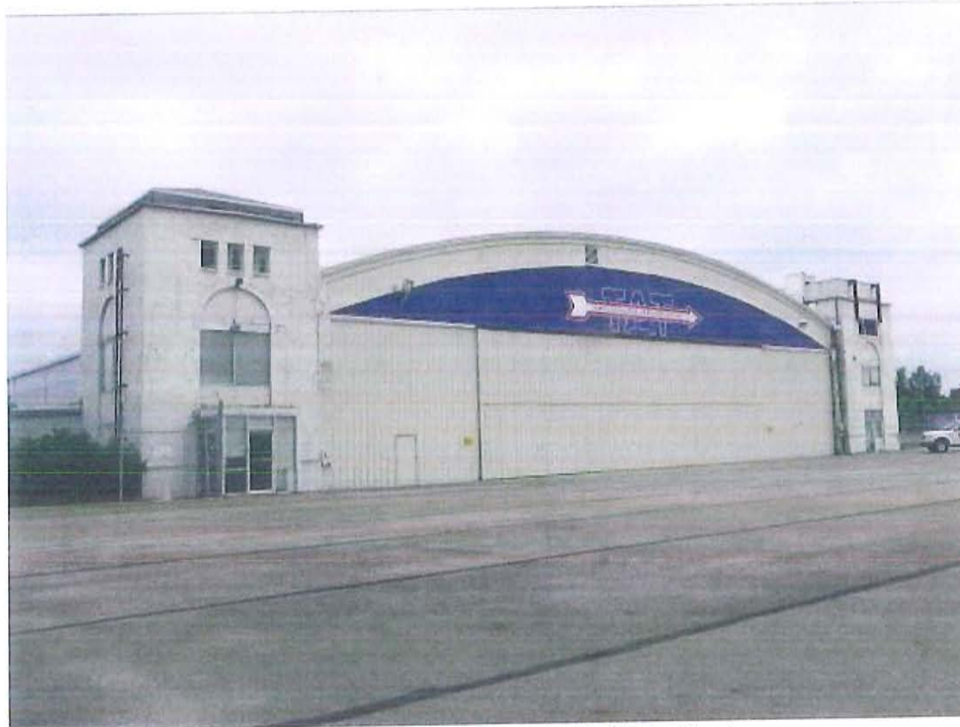
12. TAT Hanger, west elevation, looking southeast
