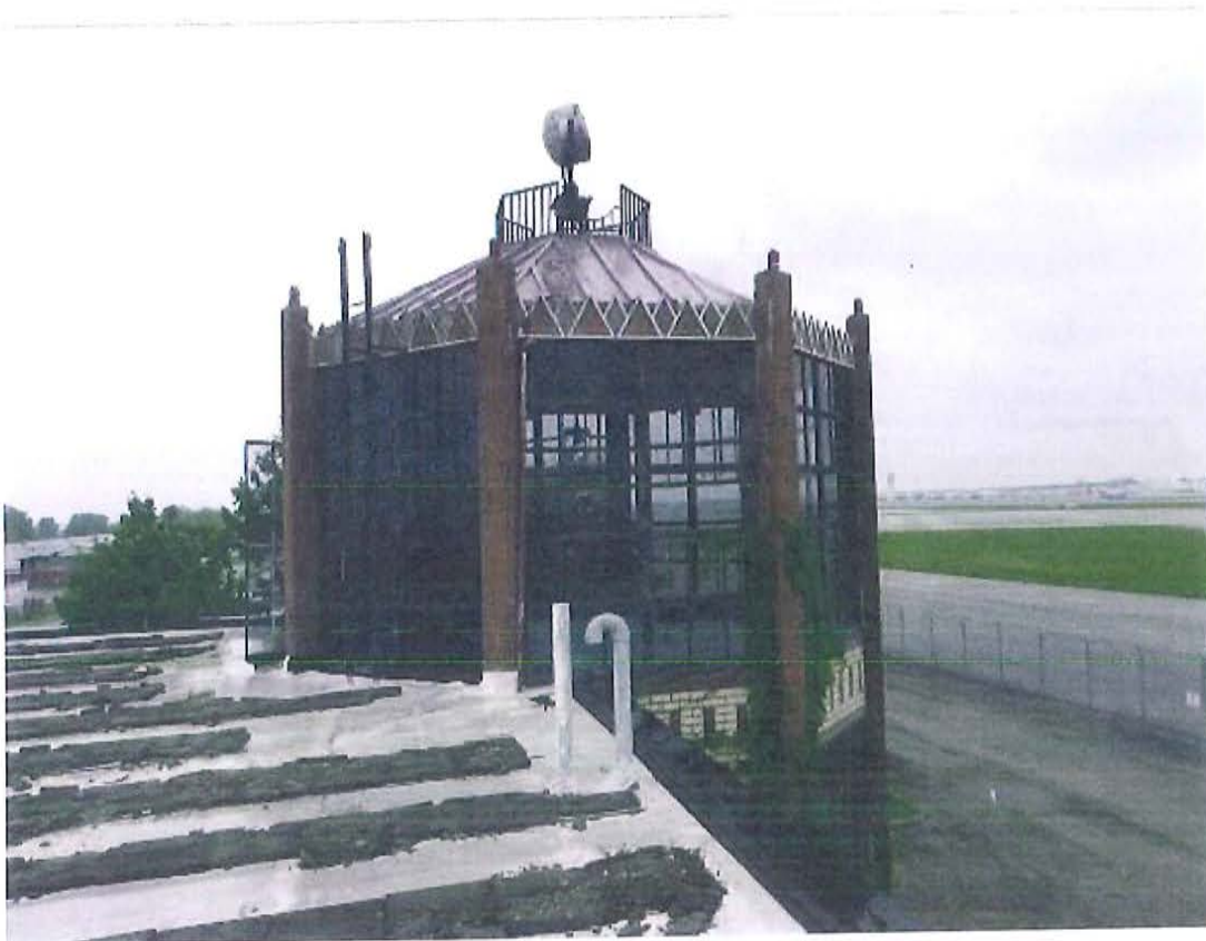
11. Passenger Terminal, tower and roof, looking west
