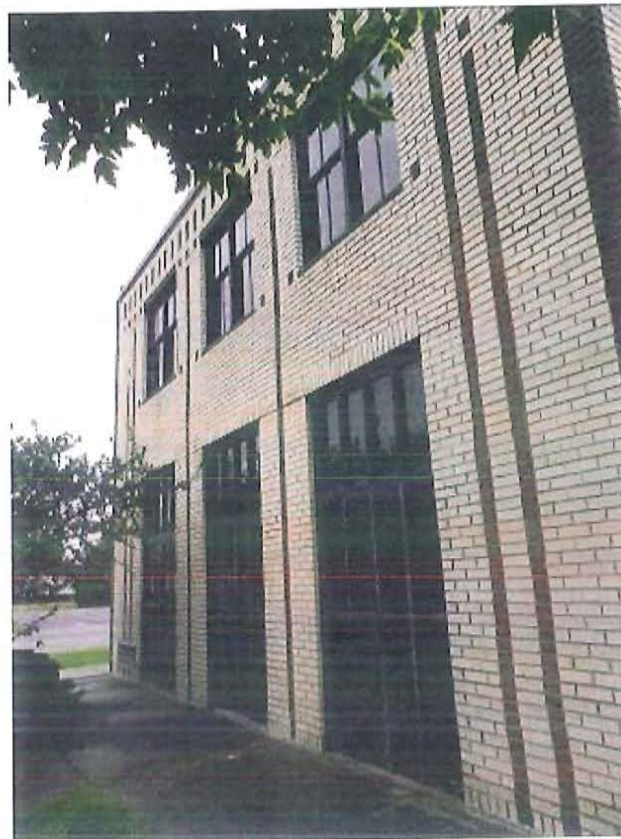
4. Passenger Terminal, east elevation, looking south
