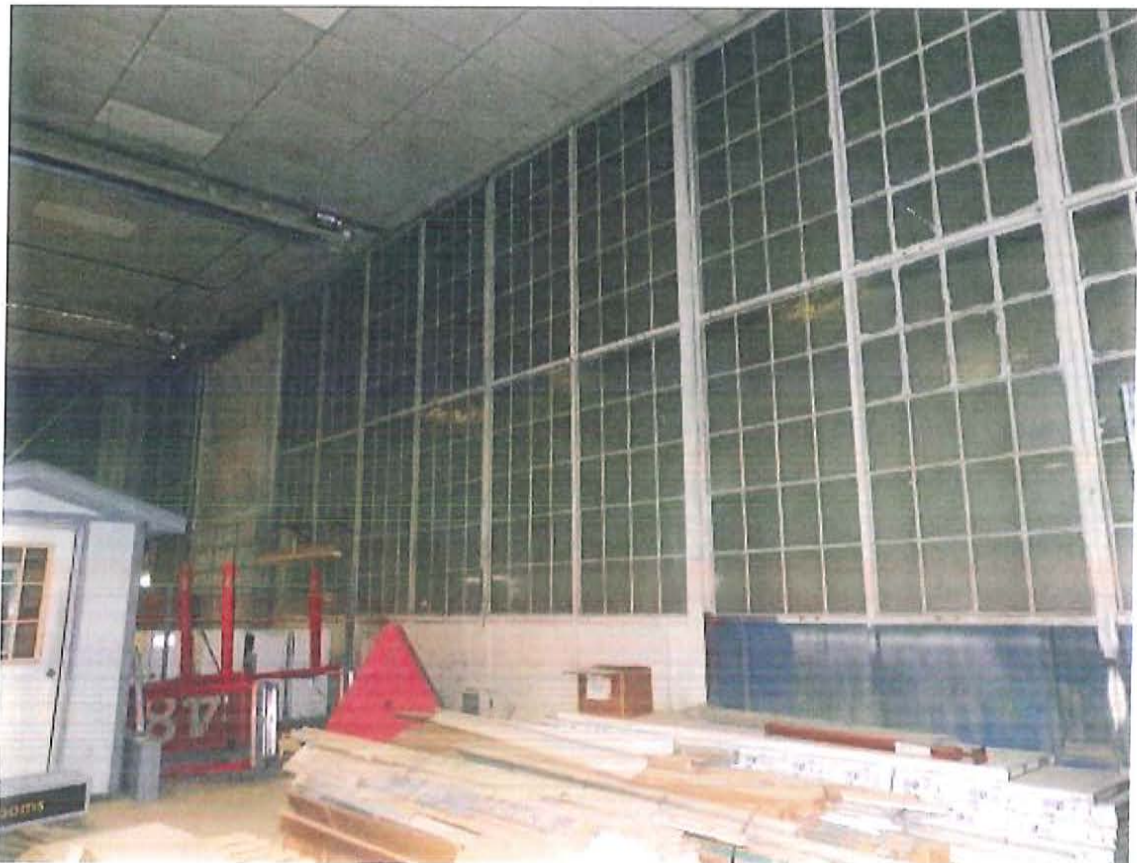
18. TAT Hanger, 1 st floor, original windows
