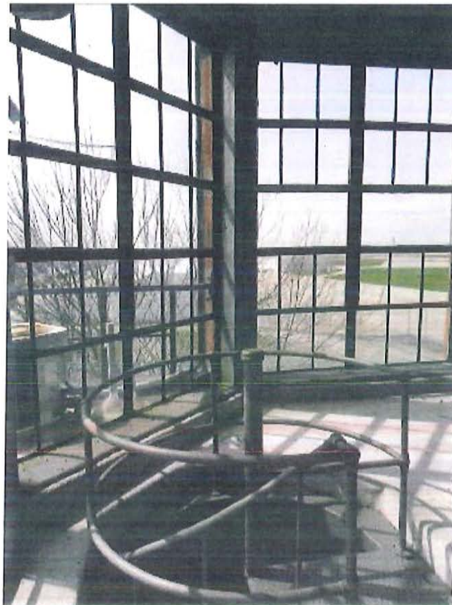
10. Passenger Terminal, 3 rd floor, looking west
