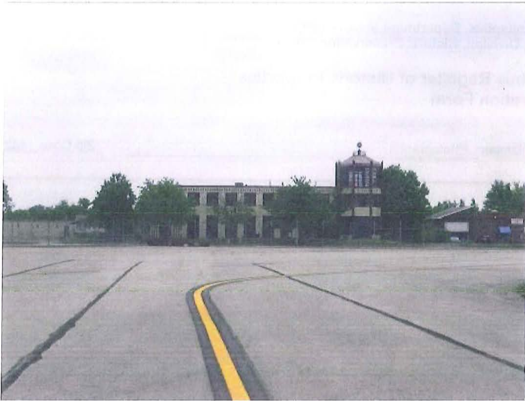
1. Passenger Terminal, view from the TAT Hangar, looking south.
