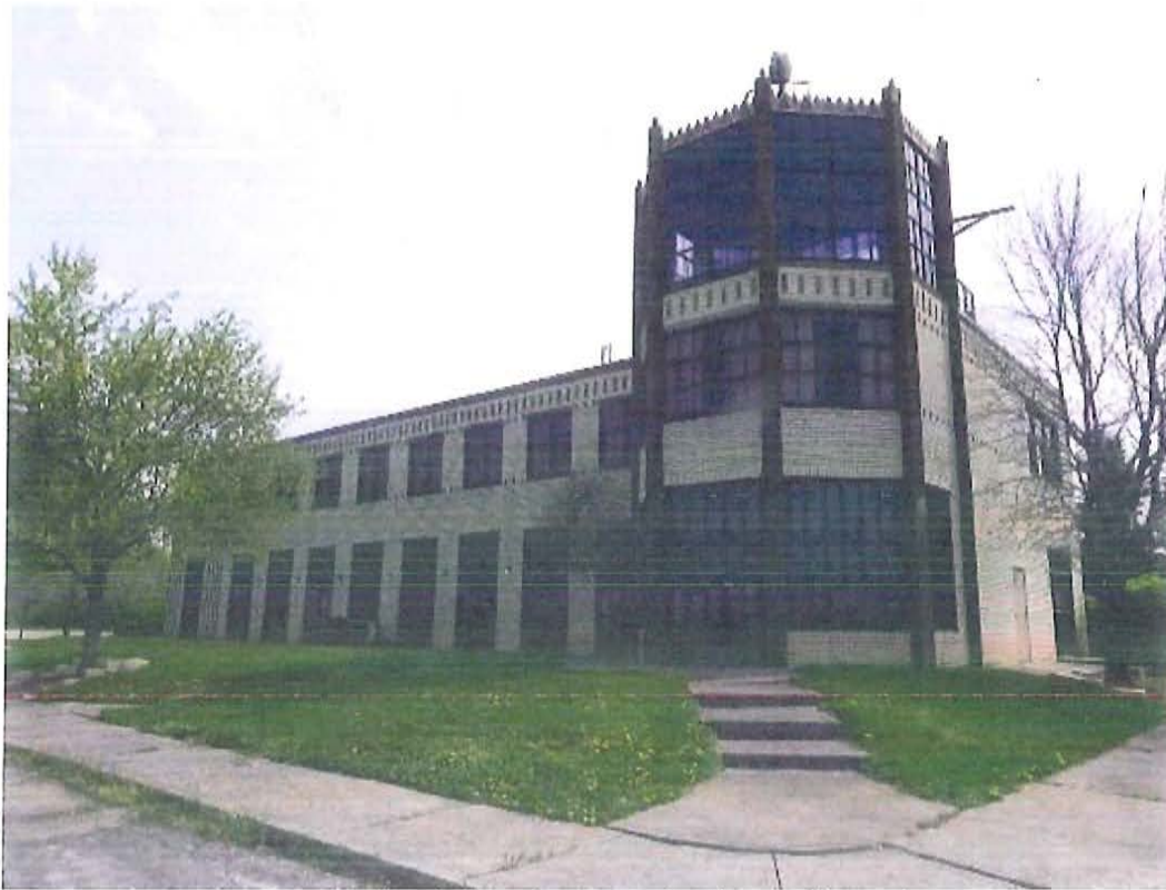
2. Passenger Terminal, north and west elevations, looking southeast
