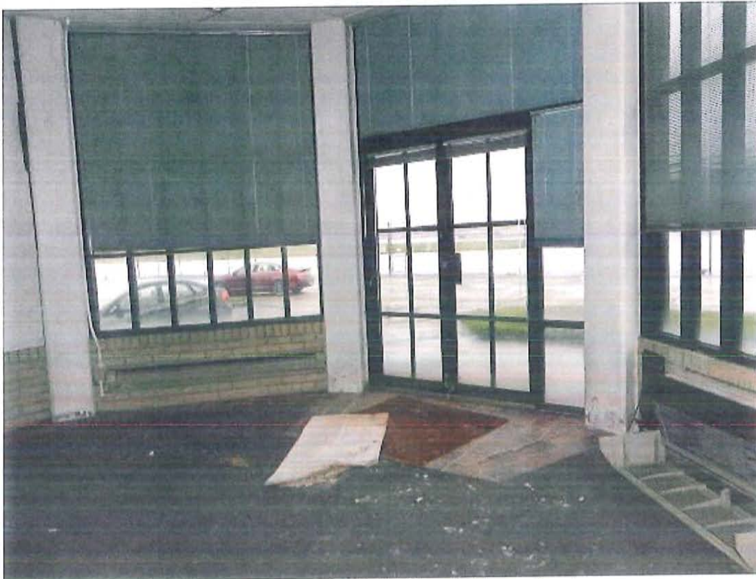
8. Passenger Terminal, 1 st floor, looking northwest
