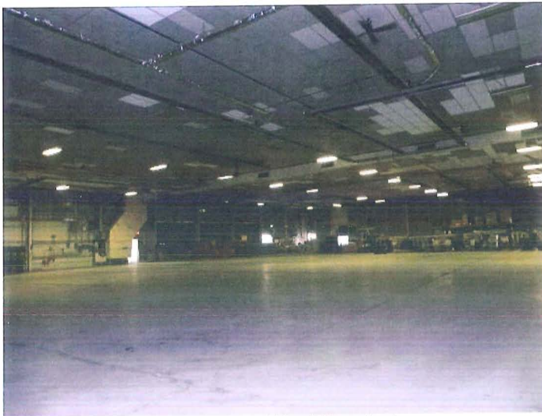
16. TAT Hanger, 1 st floor, looking northwest
