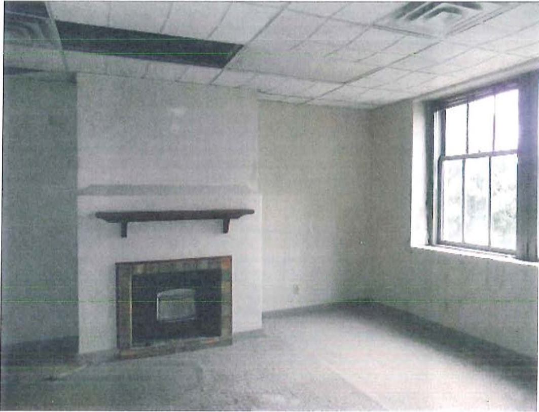
9. Passenger Terminal, 2 nd floor, looking southeast
