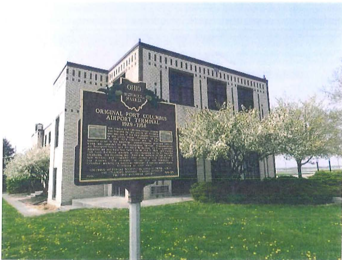
5. Passenger Terminal, east and south elevations, looking northwest
