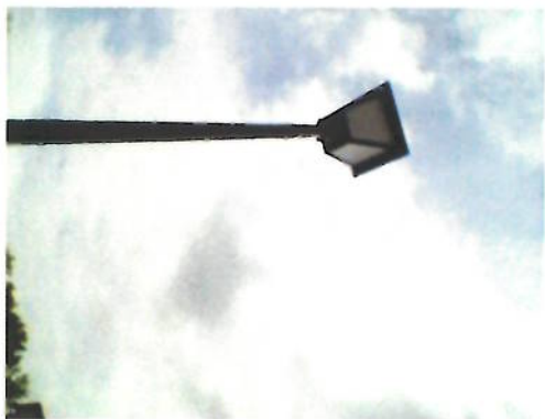
150 WATT MH RLB BLACK FIBERGLASS POLE DIRECT BURIAL
