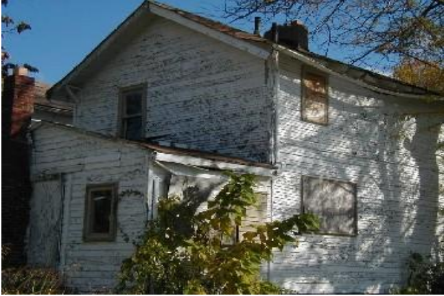
Rear of Fourth Street Double (no address posted)
