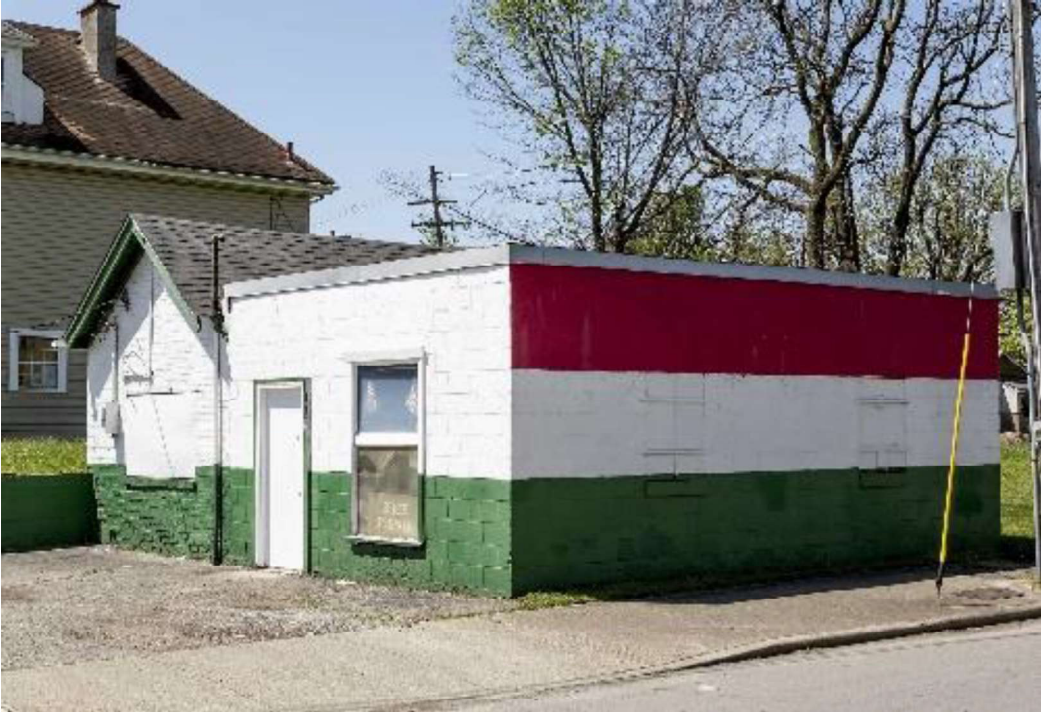
View Facing Northeast Corner of Building
