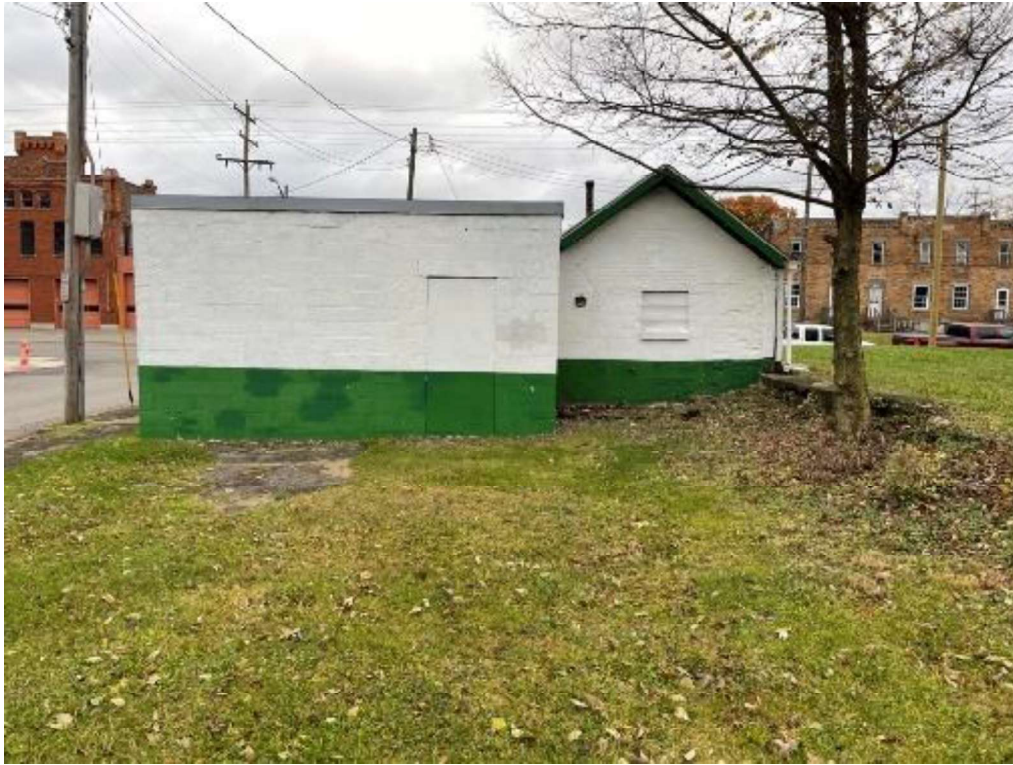
West (Rear) Elevation – Original Building with Gabled Roof on Right; Flat-Roofed Addition on Left
