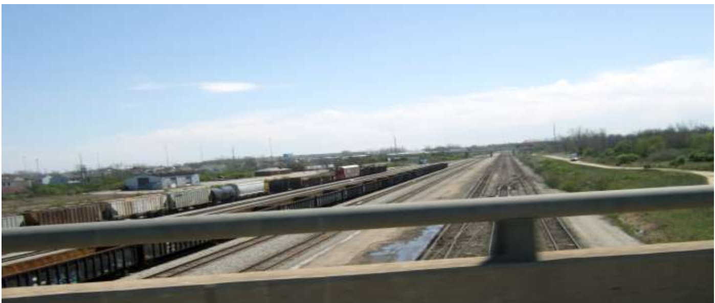
The Buckeye Rail Yard looking south on Trabue Road
