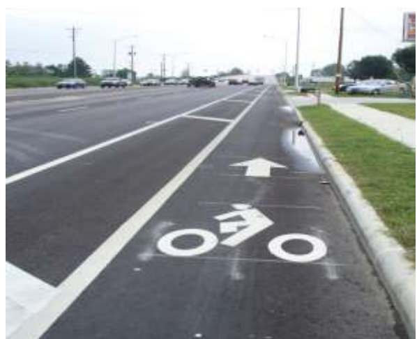
New improvements to Roberts Road, including bike lanes
