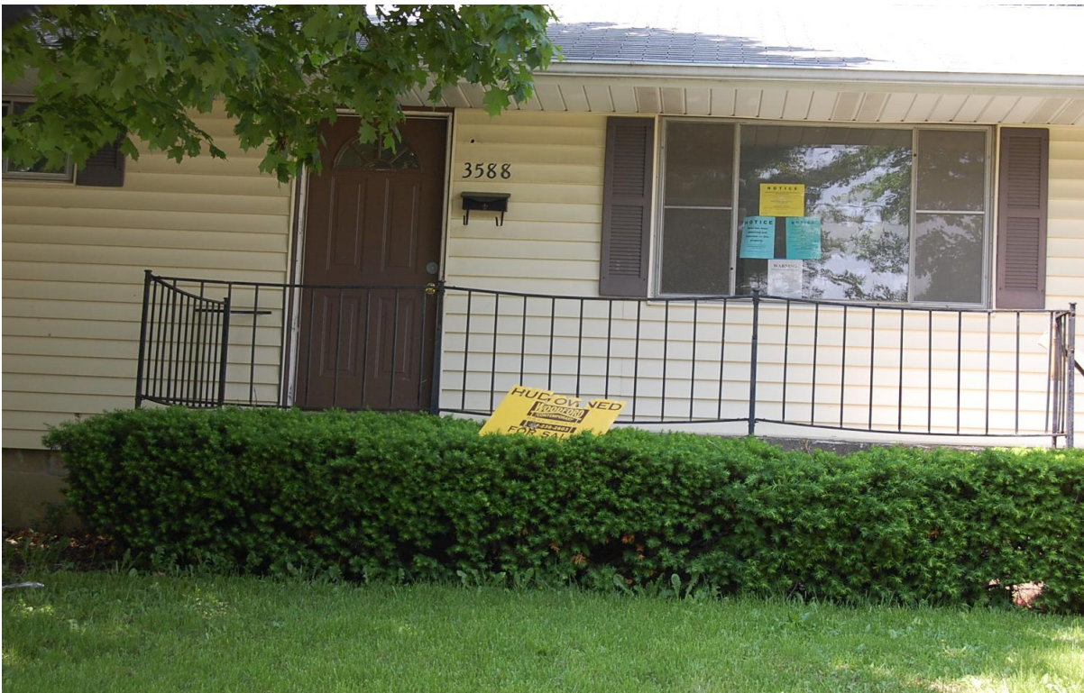
1466 Aven (note falling gutters)
