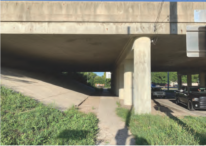
EXISTING CONDITIONS: RICH STREET & TOWN STREET UNDERPASS
