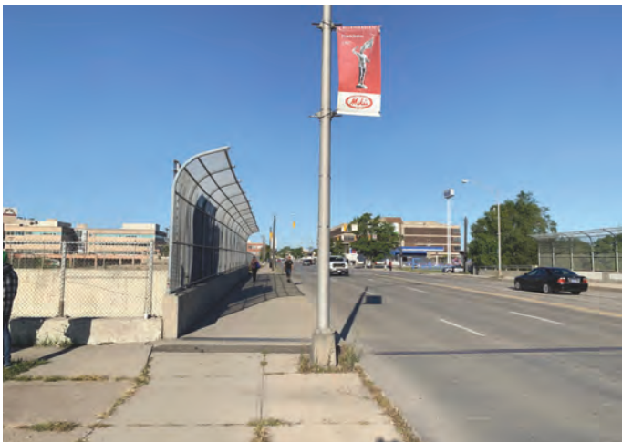
EXISTING CONDITIONS: WEST BROAD STREET OVERPASS
