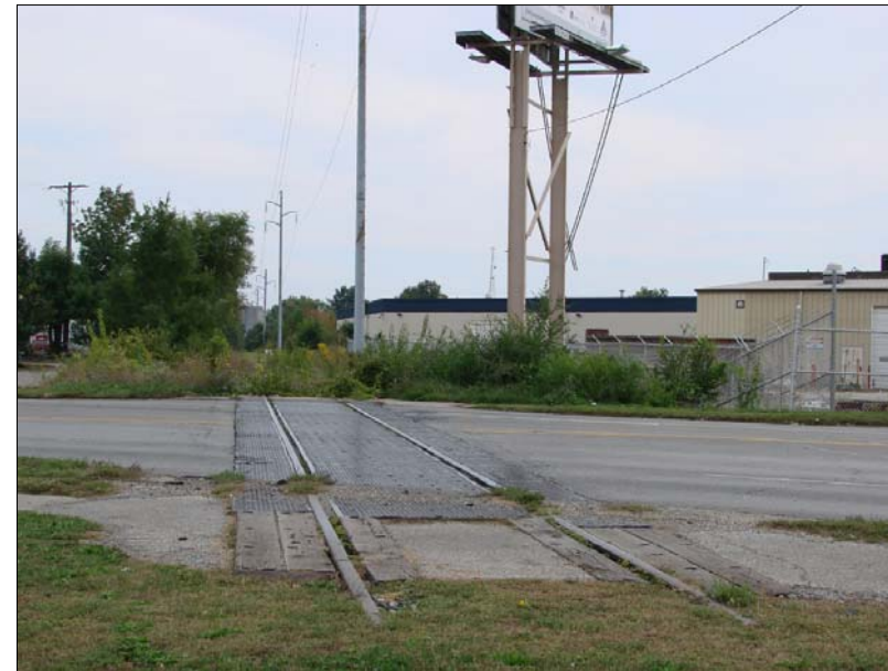
The partially-abandoned railroad right-of-way looking south from Livingston Avenue
