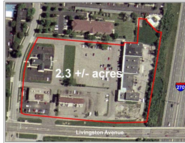
Aerial view of the York Plaza site.
