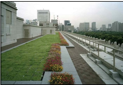
Green roofs are strongly encouraged as a way of managing stormwater and reducing microclimate impacts on buildings.
