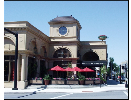
The I-670 Cap was highly successful at bridging the "gap" between the Short North and Downtown/North Market/Arena Districts, while also creating a unique dining and entertainment destination.
