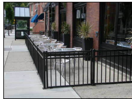
Commercial patios for restaurants and bars serving alcohol must meet fencing requirements of the Ohio Department of Commerce, Division of Liquor Control.
