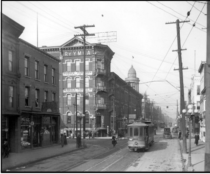
High Street in 1914 where the I-670 Cap has been constructed.
