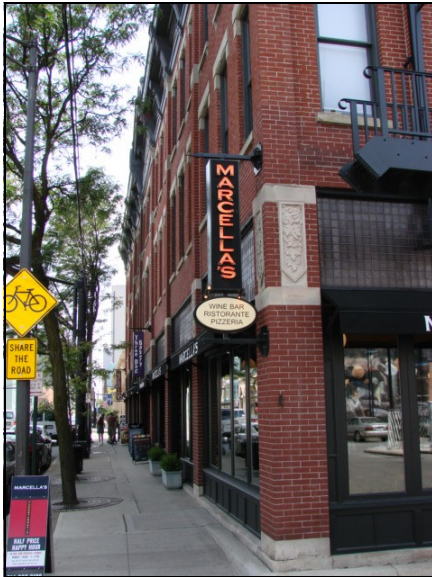
The Yukon Building is an example of a structure cited with a zero-foot setback off of the right-of-way of High Street.
