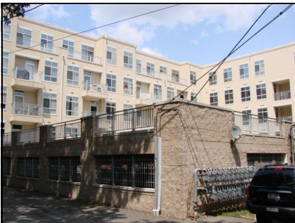
Parking structures should be integrated into projects and hidden behind principal buildings.
