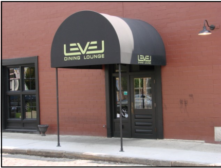
Awnings placed at a building entrance, perpendicular to the building elevation, are considered to be entrance canopies.
