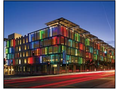
Parking garages can serve as significant architectural statements, as in this Santa Monica, California, public garage ...
