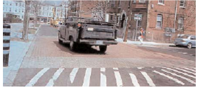
A raised intersection to calm traffic
