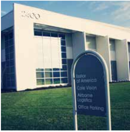
Light industrial facilities can be attractive and have positive impacts on surrounding neighborhoods.
