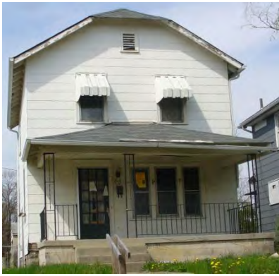
638 E GATES ST 010-003610
