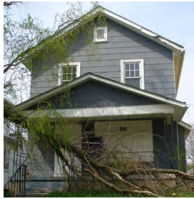
642 E GATES ST 010-003609
