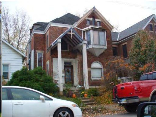
83 E GATES ST 010-049247
