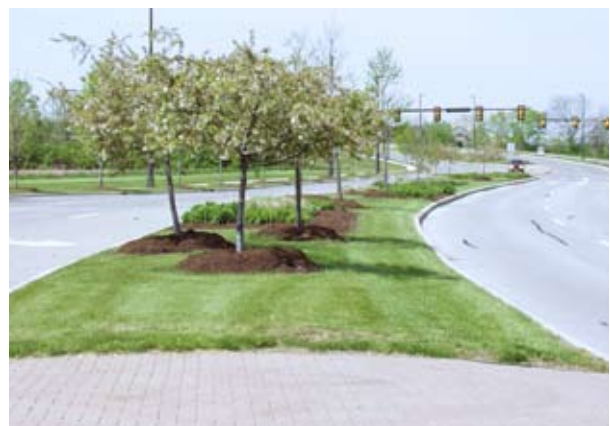
Five-lane road with landscaped median Two moving lanes of traffic in each direction with one center turn lane. Landscaped median located where the turn lane is not necessary.
