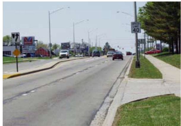
Five-lane road Two moving lanes of traffic with one center turn lane.
