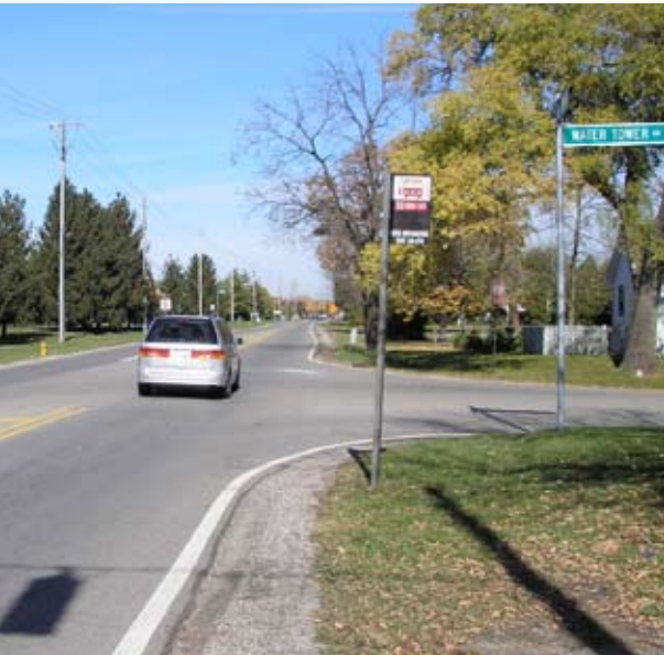
Collector road without sidewalks or safe place to stand at bus stop.
