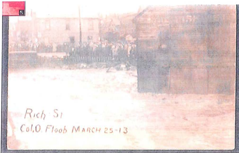
Figure 1: Rich Street (flood), Franklinton, Ohio, March 25, 1913. Columbus Metropolitan Library
