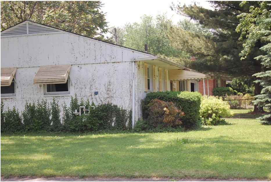
3588 Bolton (note vacancy signage in the windows- HUD owned)
