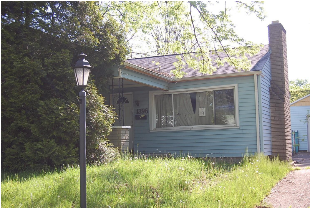
1306 Zettler (note vacancy signage in windows)
