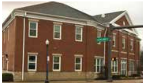
CMHA Office Building Located at East 11th Avenue & Cleveland Avenue
