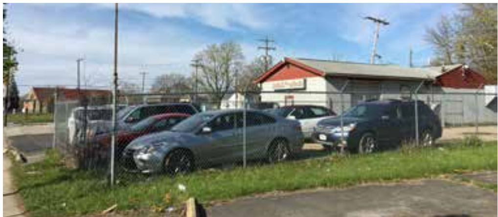
Body Shop on Cleveland Avenue Representing a Common Commercial Use Found Along the Commercial Corridors in South Linden
