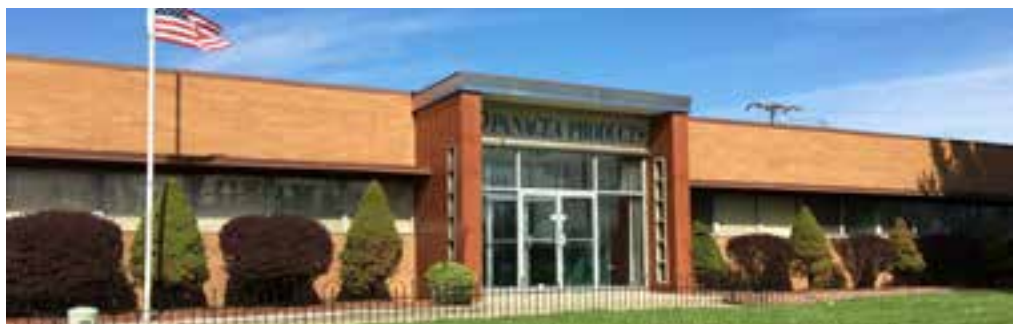
Light Industrial Building on the West Side of Joyce Avenue
