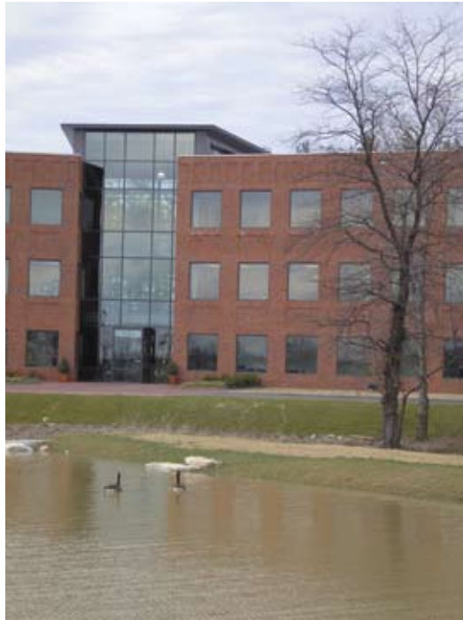
Three-story office building
