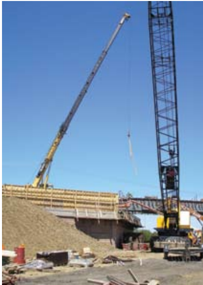
Current work on US 33 Ebright Rd. overpass (2007)
