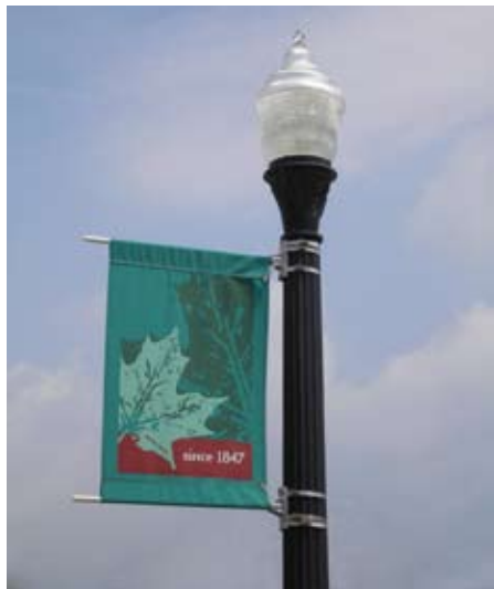
Capped post lighting fixture
