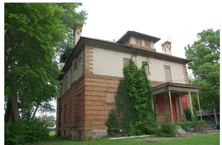
4. South and east elevations, looking west
