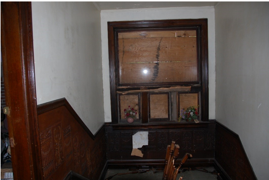
15. 2 nd floor, formal stairs, looking north
