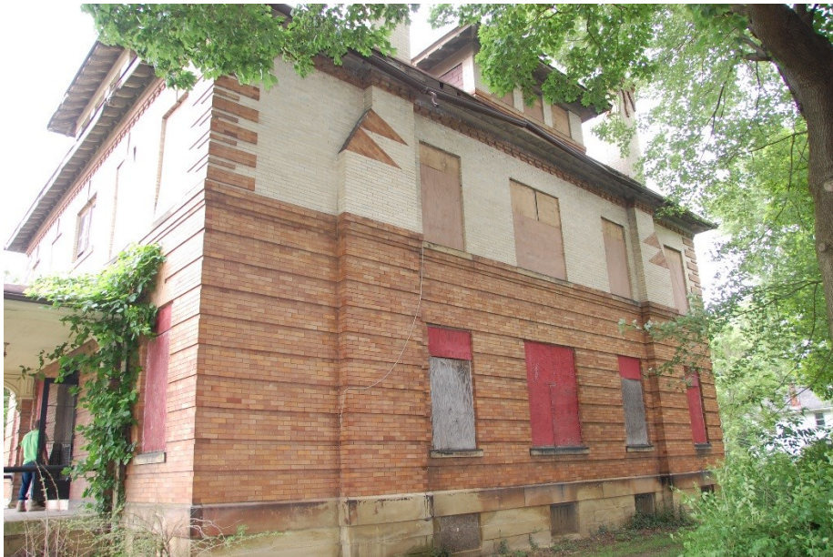
3. Façade and south elevation, looking northeast
