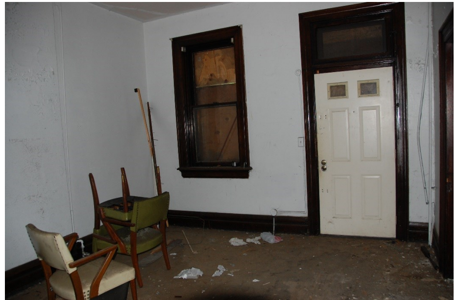
14. 1 st floor, looking northeast
