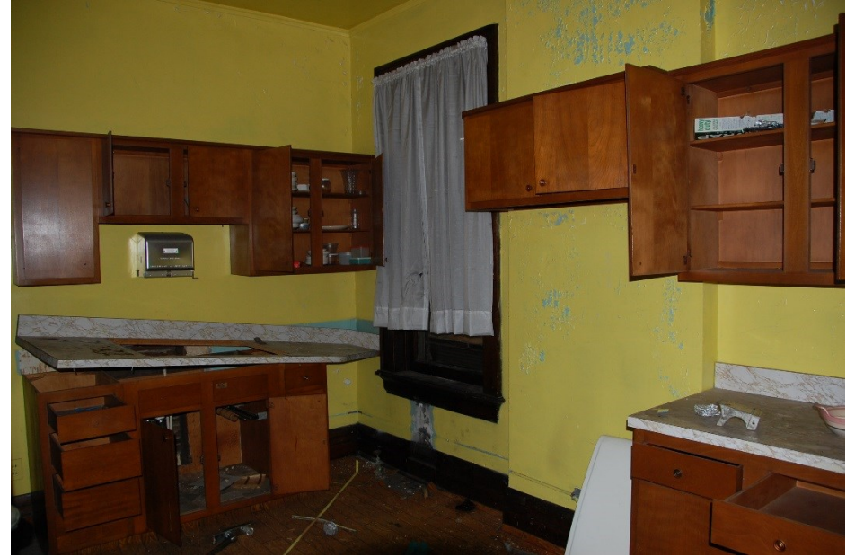
18. 2 nd floor, looking northwest
