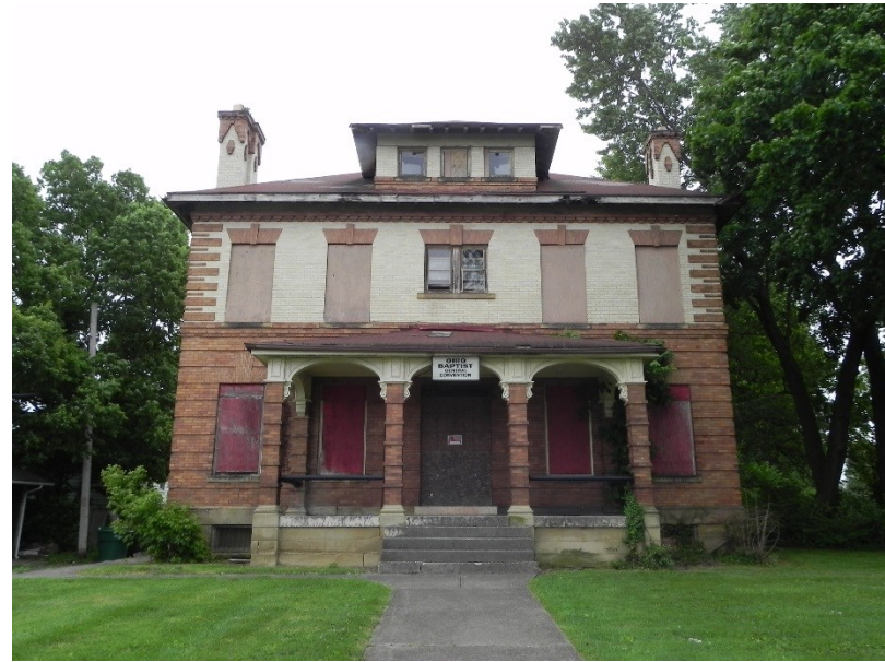
2. Façade, looking east
