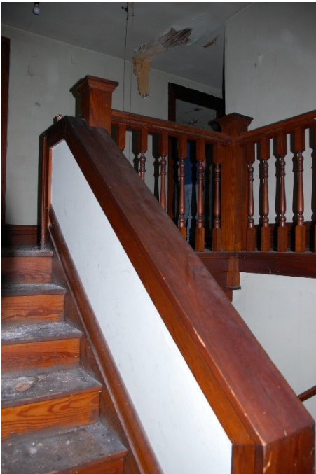
19. 3 rd floor, servants' stairs, looking southwest
