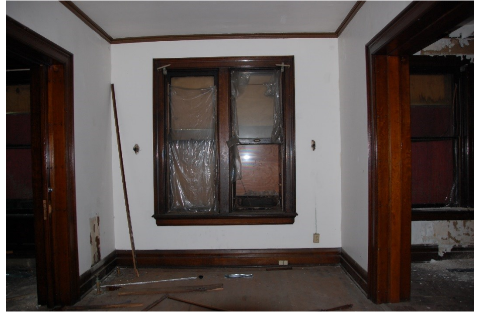
10. 1 st floor, looking south
