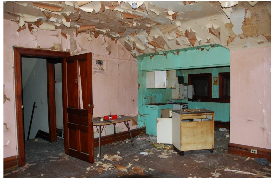
20. 3 rd floor, looking northeast
