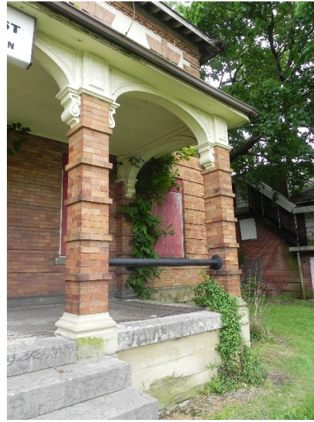
6. Porch detail, looking southeast
