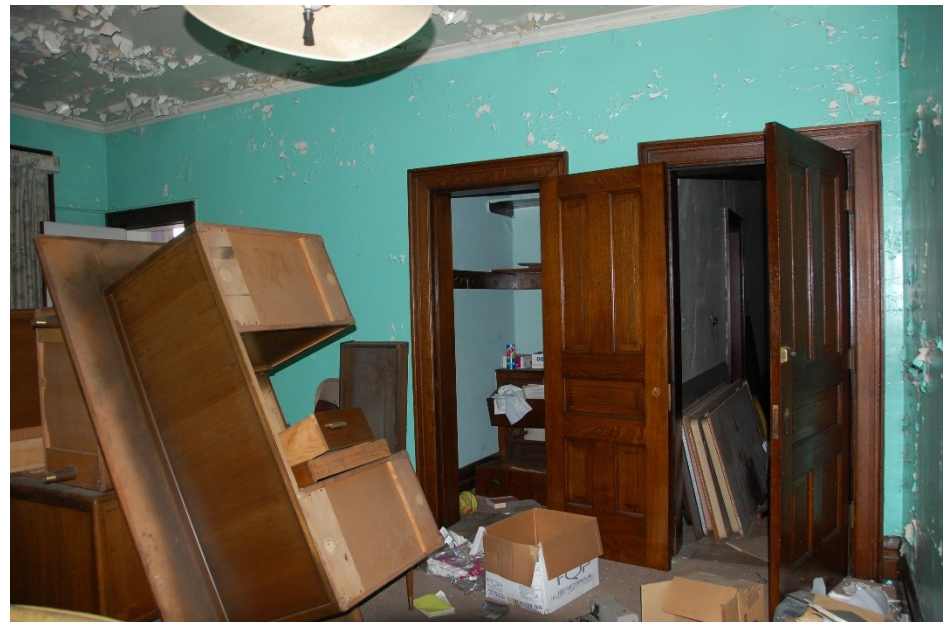
16. 2 nd floor, looking northwest
