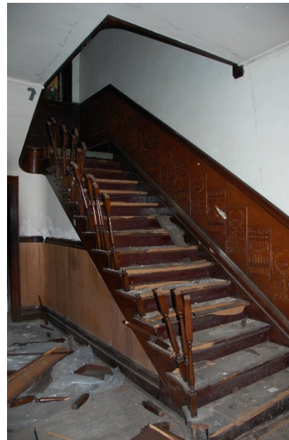
8. 1 st floor, formal stairs, looking northeast
