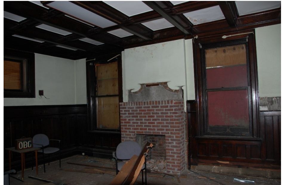
12. 1 st floor, dining room, looking southeast
