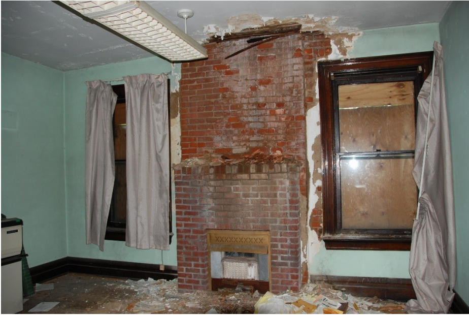
17. 2 nd floor, looking southeast
