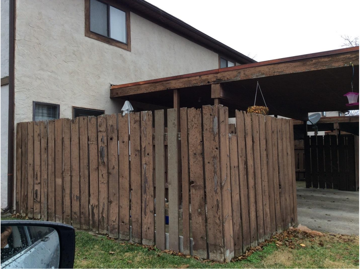
1214 Olde Henderson Square
