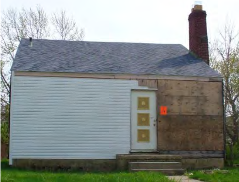
659 E GATES ST 010-023181
