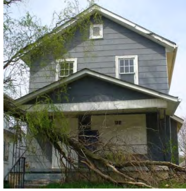
642 E GATES ST 010-003609
