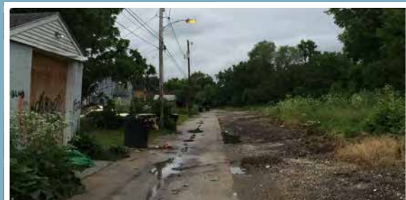
ALLEYS IN DISREPAIR
