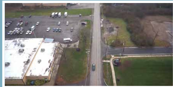
HARMON AVENUE CORRIDOR
