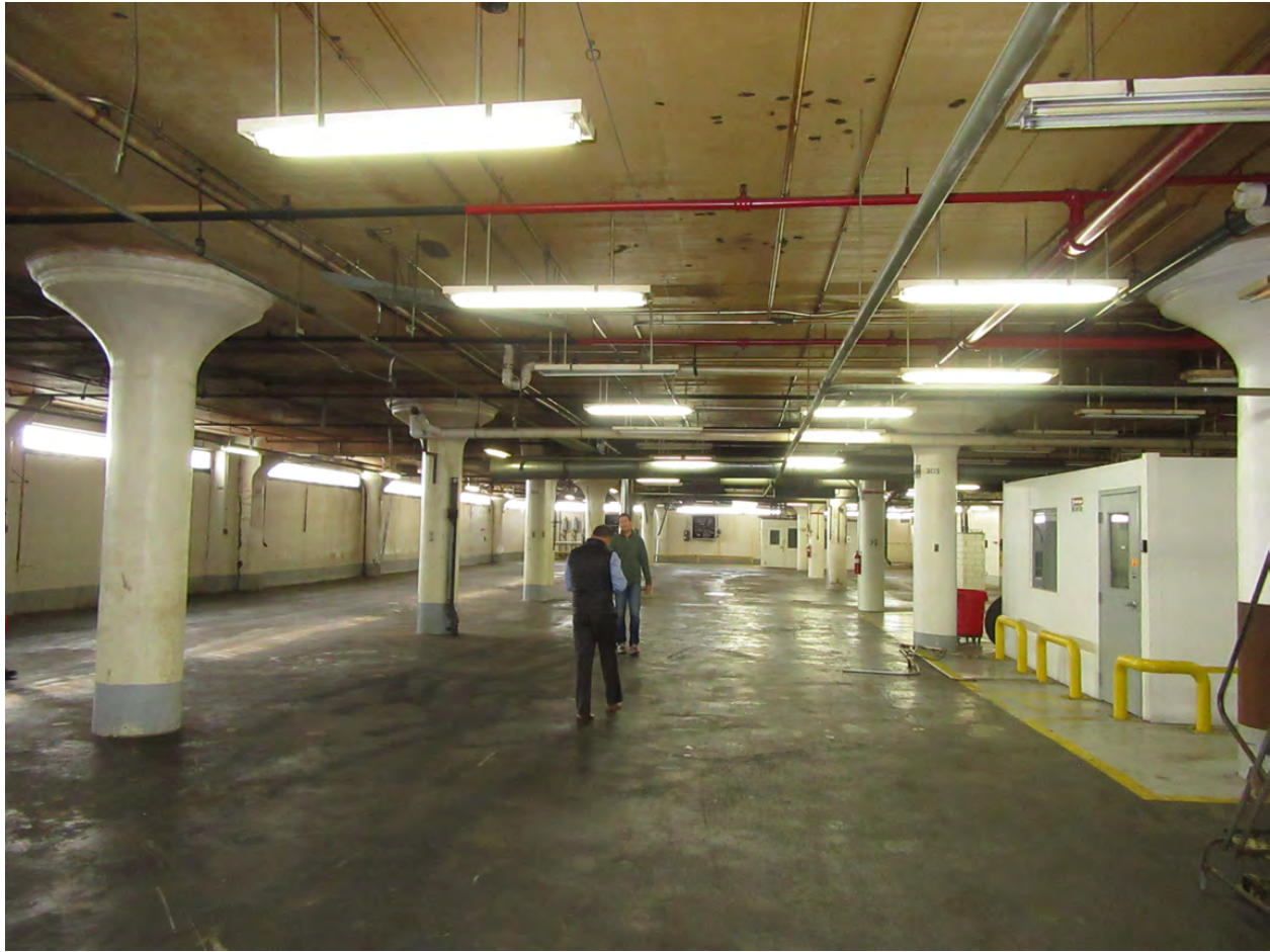
Photo 8 – Third floor, typical interior in c.1918 addition, camera facing south
