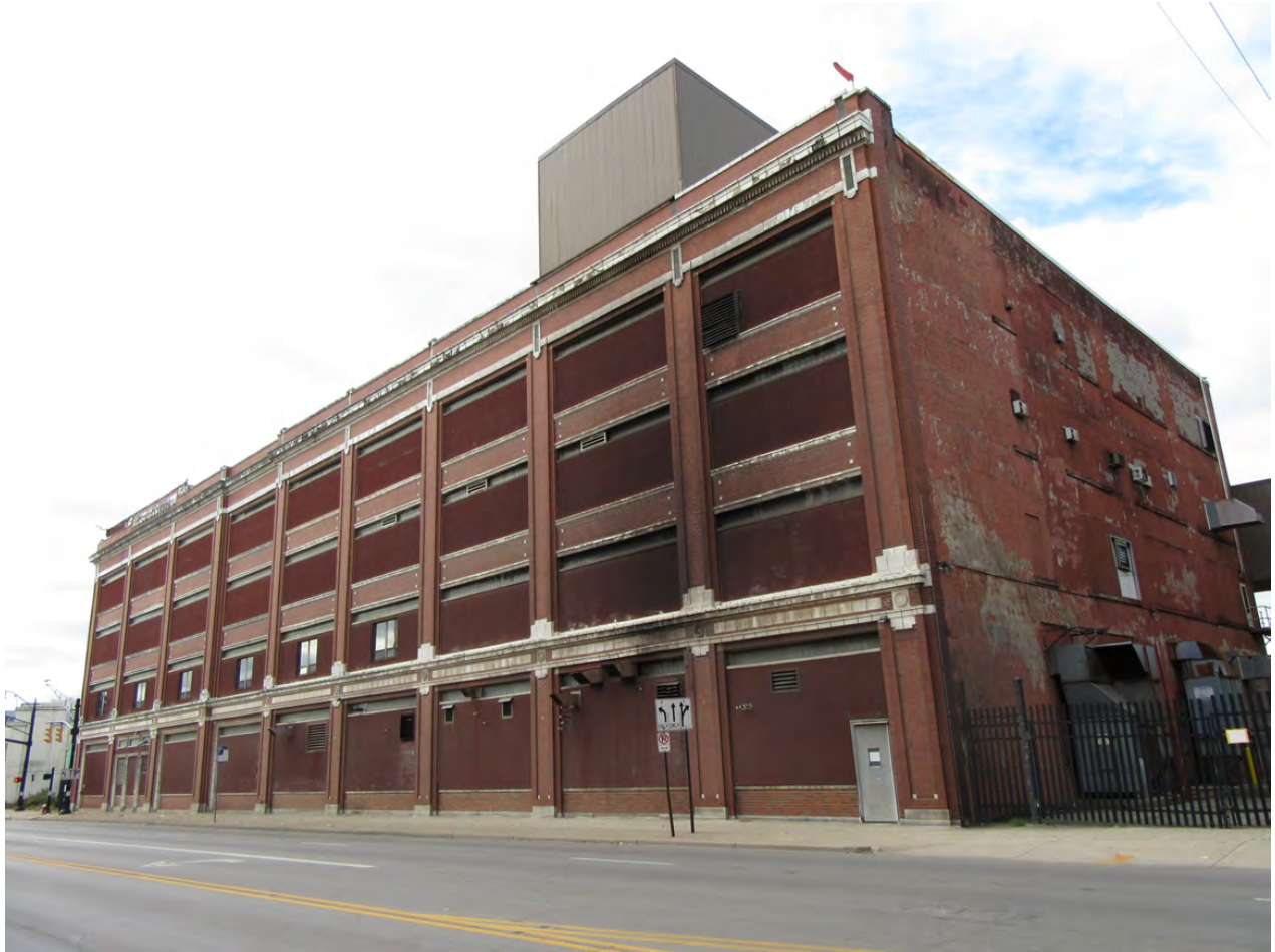
Photo 2 - Northeast oblique, camera facing southwest
