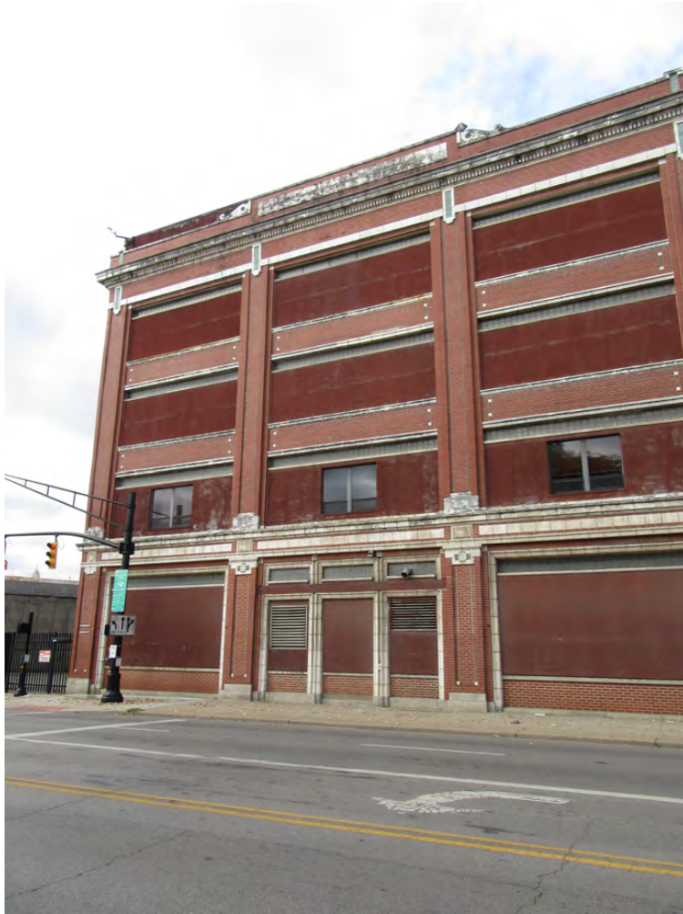
Photo 3 - East façade, south end, camera facing southwest
