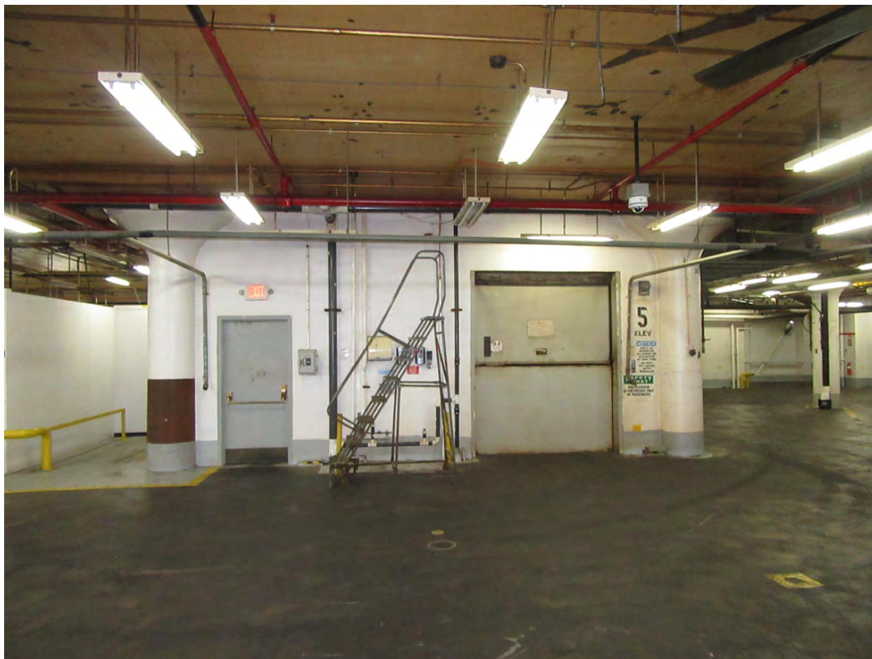
Photo 9 – Third floor, typical stair/elevator core in c.1918 addition, camera facing west
