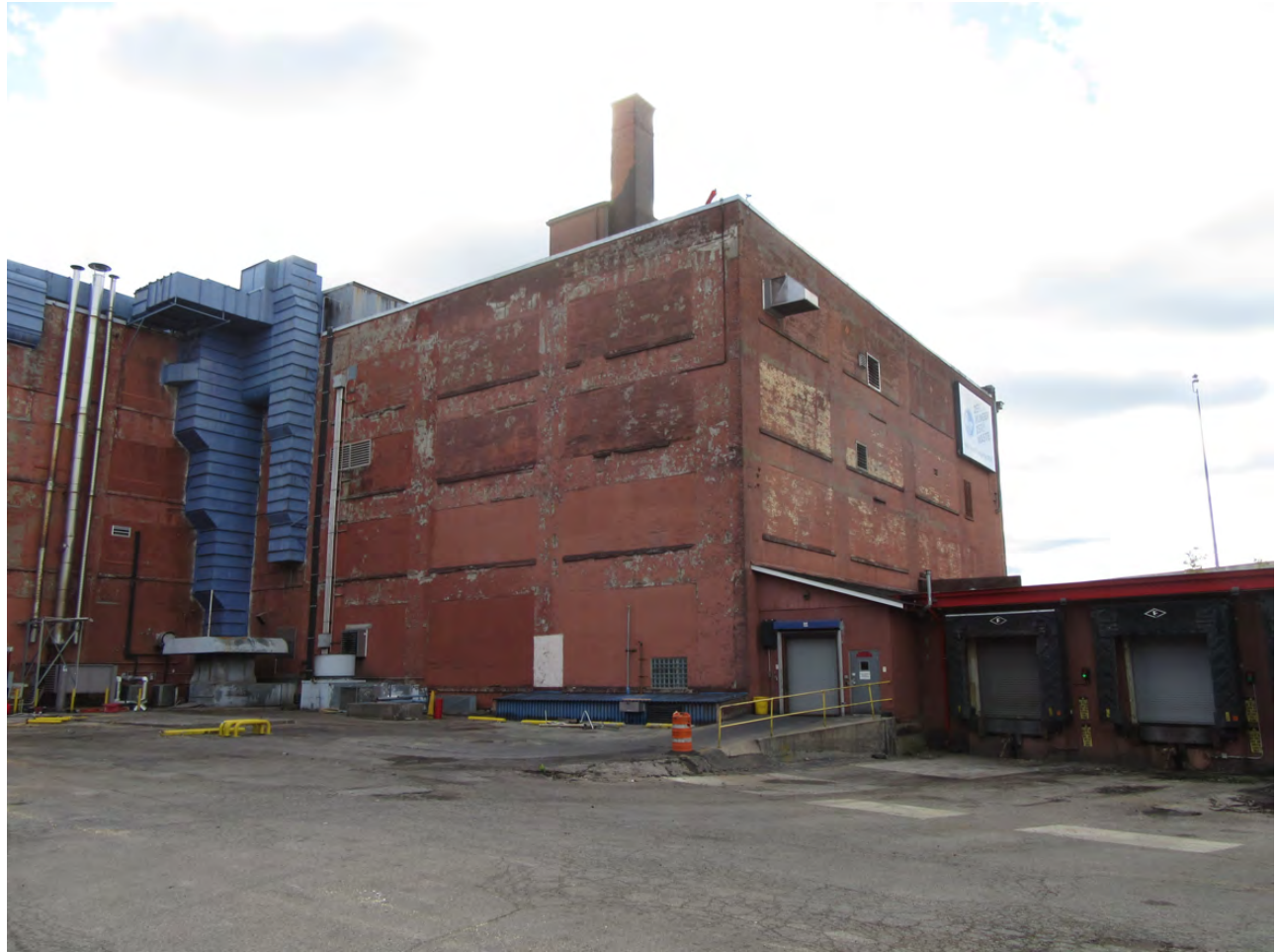
Photo 5 – Northwest oblique, original section, camera facing southeast
