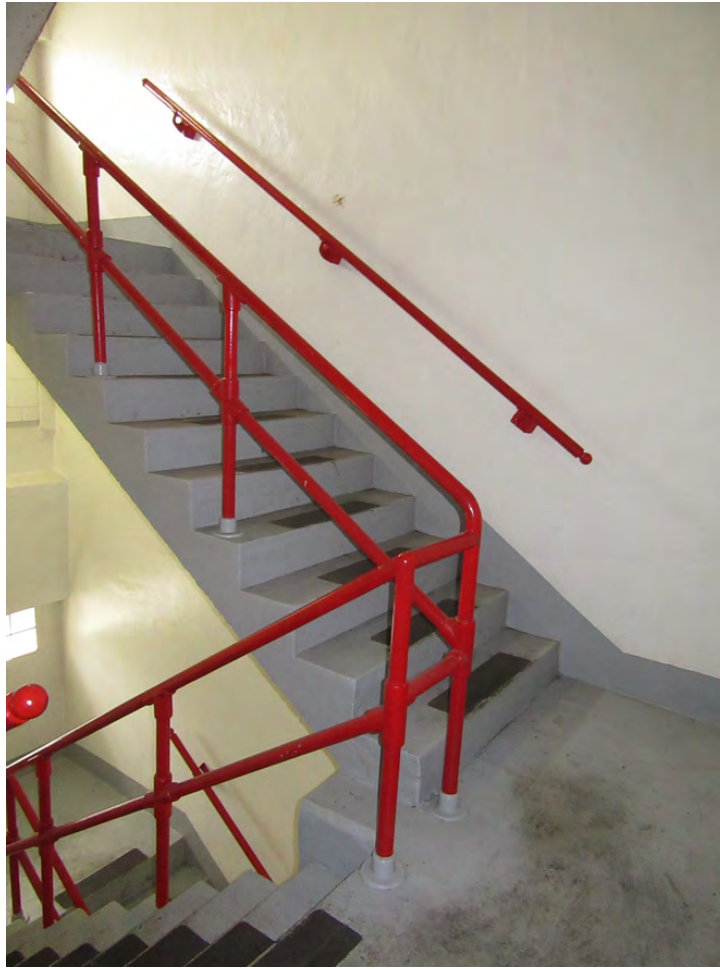
Photo 10 – Typical utilitarian stairs, camera facing southwest
