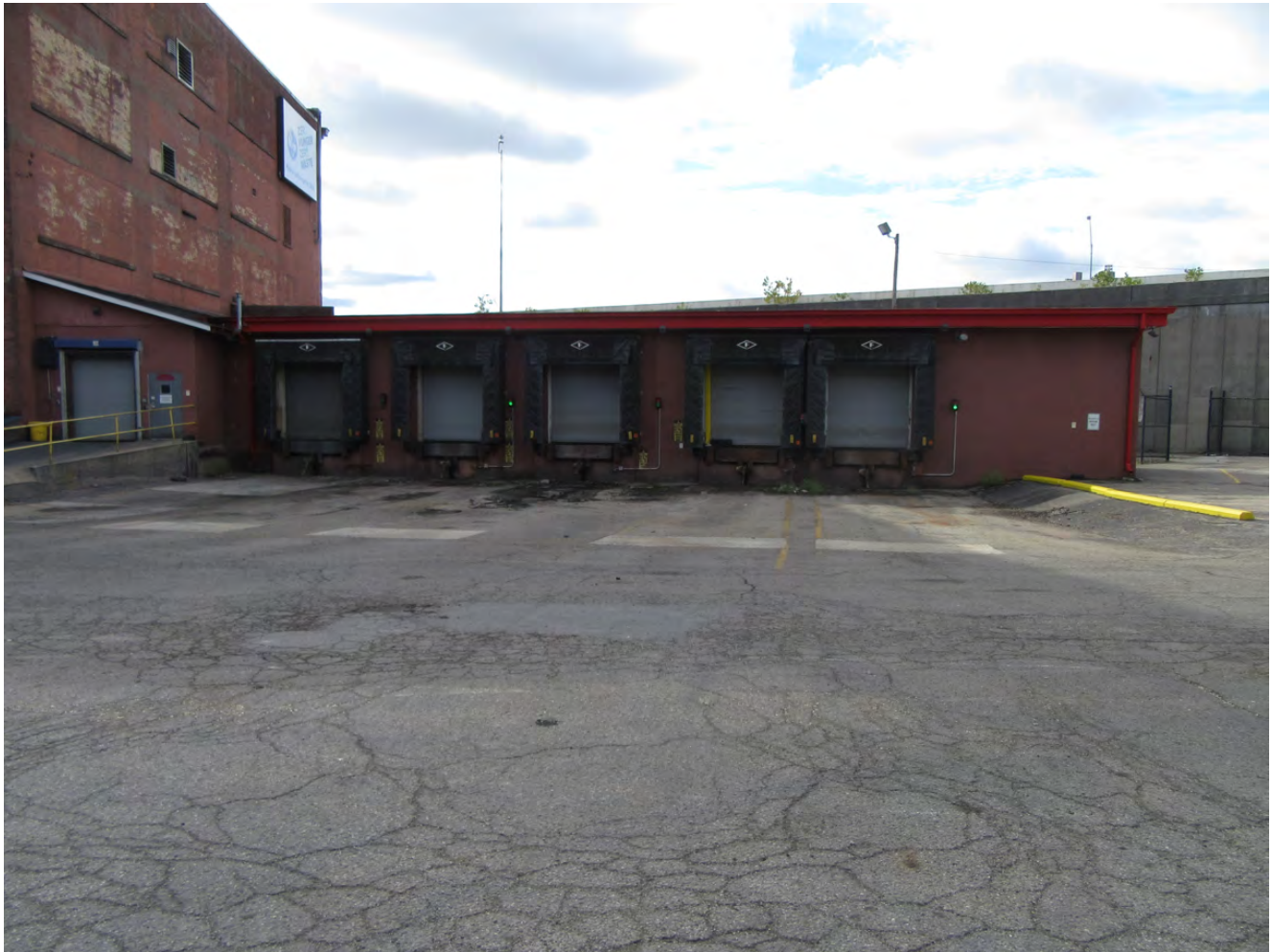
Photo 6 – North elevation, non-historic truck dock addition, camera facing south
