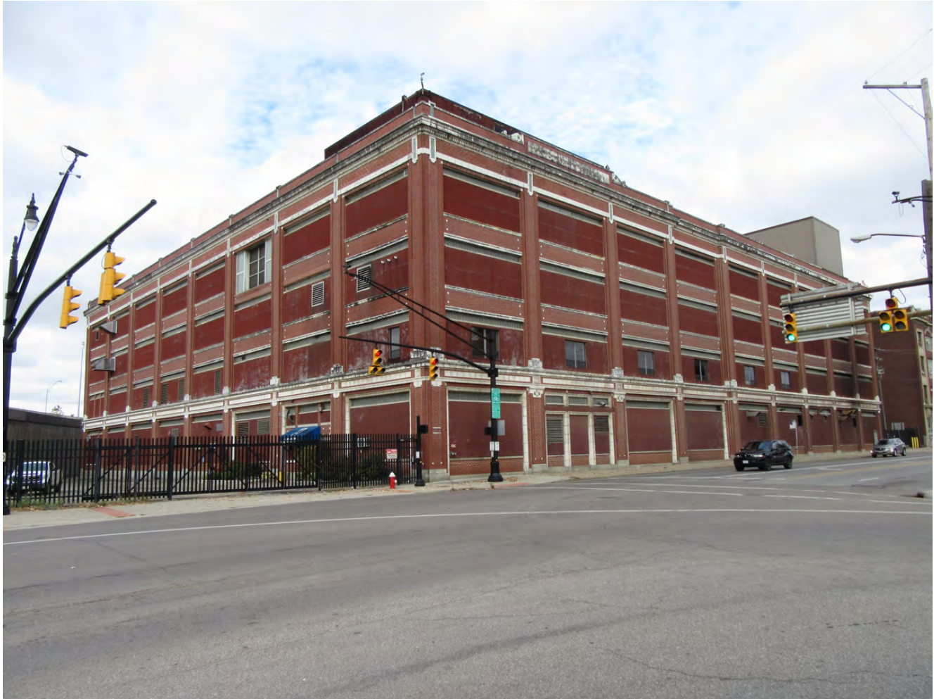
Photo 1 - Southeast oblique, camera facing northwest
