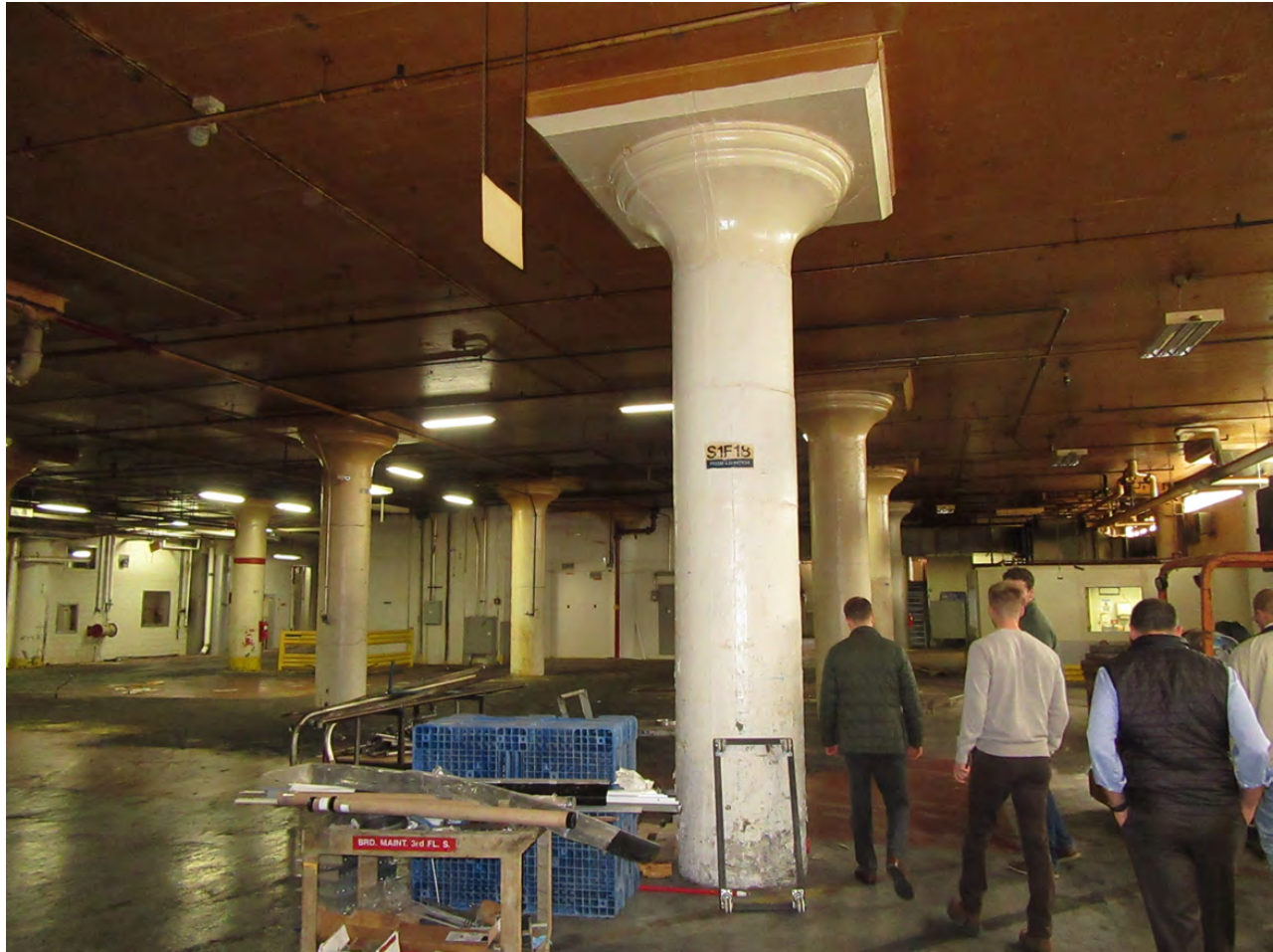
Photo 7 – First floor, typical interior in original section, camera facing northeast
