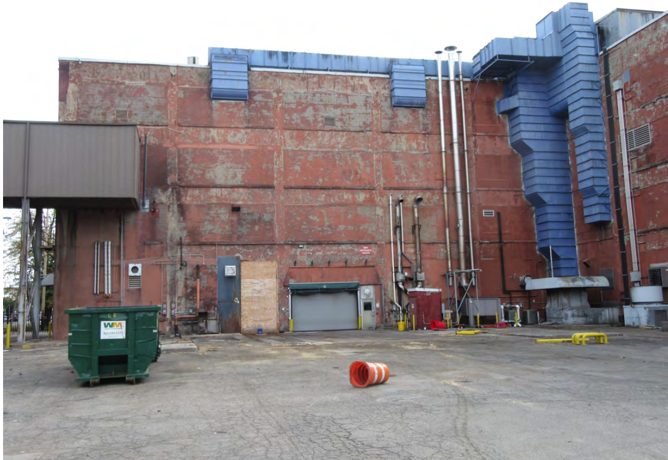
Photo 4 – West elevation, c.1918 addition, camera facing east
