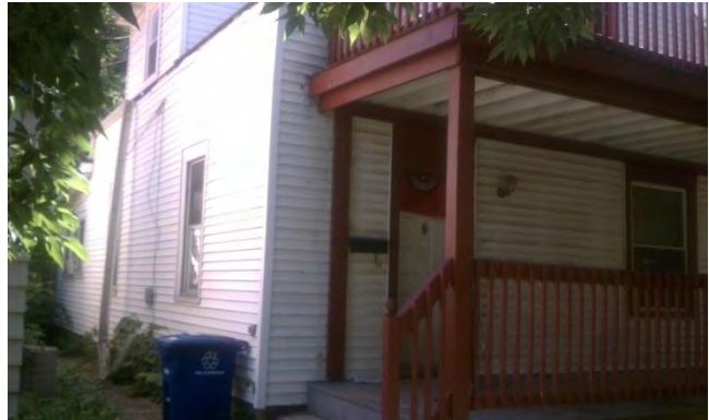
369 E GATES ST 010-003024
