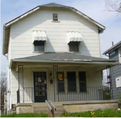
638 E GATES ST 010-003610
