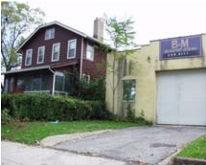
Example of inappropriate massing, Camden Avenue.
