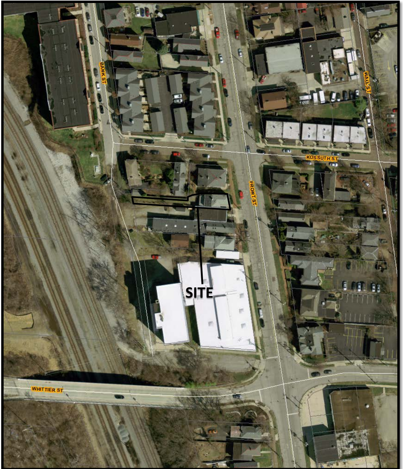
CV16-038 825 South Front Street Approximately 0.07 acres
