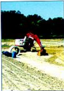
Construction site at New World Drive and Alum Creek Drive.
