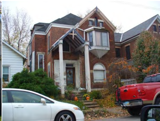
83 E GATES ST 010-049247
