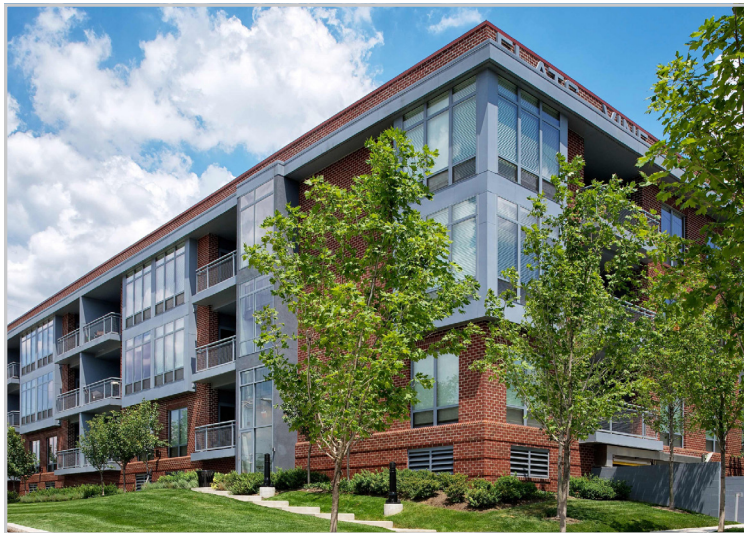
An example of a structure that places housing over podium parking.
