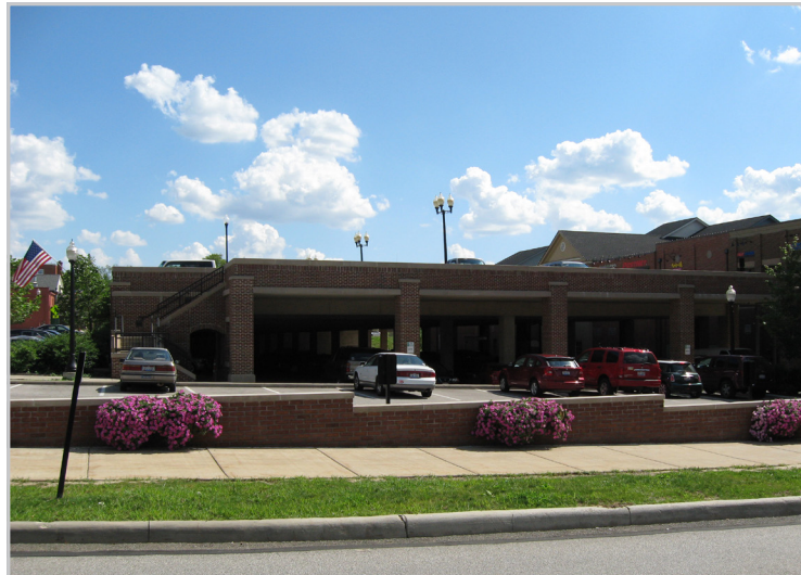
Parking example screened by landscaping and architectural features.
