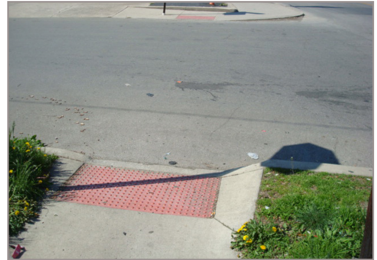
Existing curb ramps offer room for improvements to be ADA compliant.
