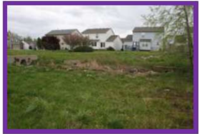
Figure 10c: Vegetation around outflow and inflow pipes at southeast corner of basin
