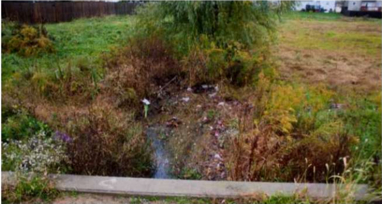
Figure 11: Basin inflow at 4:30 PM October 19, 2011, 22 hours after the photo in Figure 2 was taken and at the end of a 4.95" rain event over a 40 hour period. Records indicate that 3.85" total fell on October 19, 2011, and 1.15" fell on October 20, 2011.
