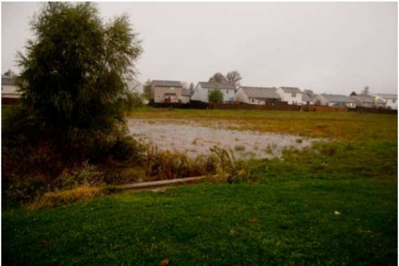
Figure 7: Basin at 6:40 PM October 19, 2011 after 3" of rain over 18 hours
