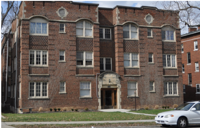
Example of a Common Entry into a Residential Multiplex
