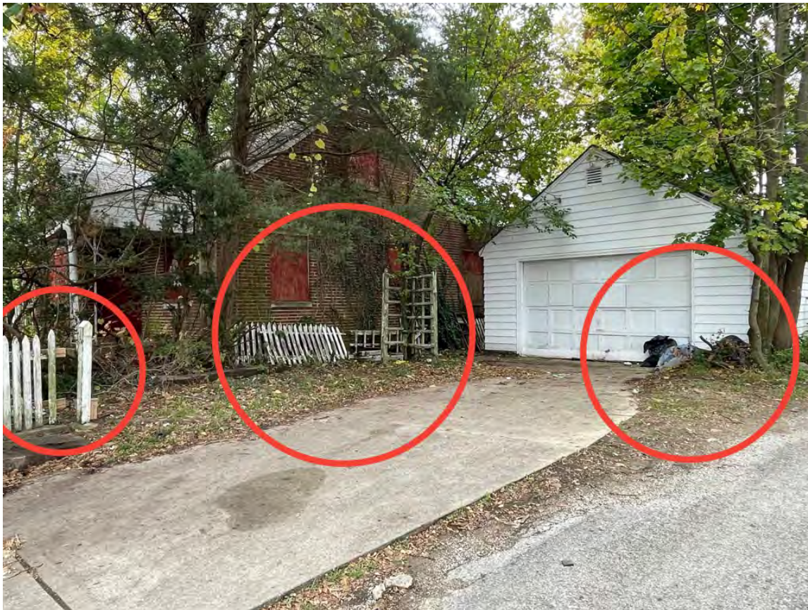
Bare exposed wood. Yard waste Damaged fencing. Solid waste/trash and debris.
