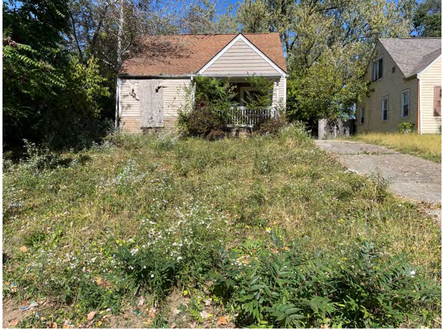
Vacant structure not boarded to code. Bare, exposed wood surfaces present on exterior. Damaged and/or missing sections of siding. Rain carriers full of debris. Missing downspout. High grass/weeds.
