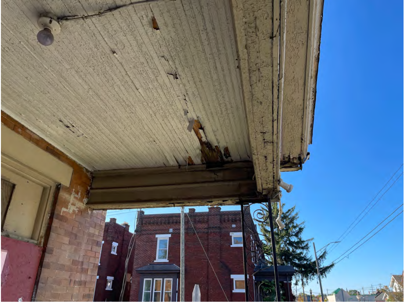
Bare and/or rotting wood surfaces on the front porch ceiling, fascia, soffits, and/or trim
