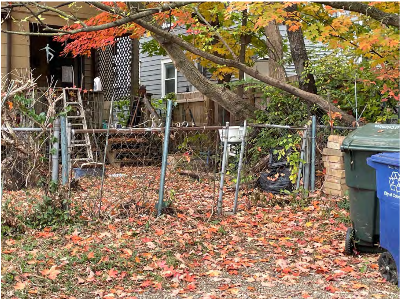
Solid waste and/or improper exterior storage of construction materials and/or miscellaneous items
