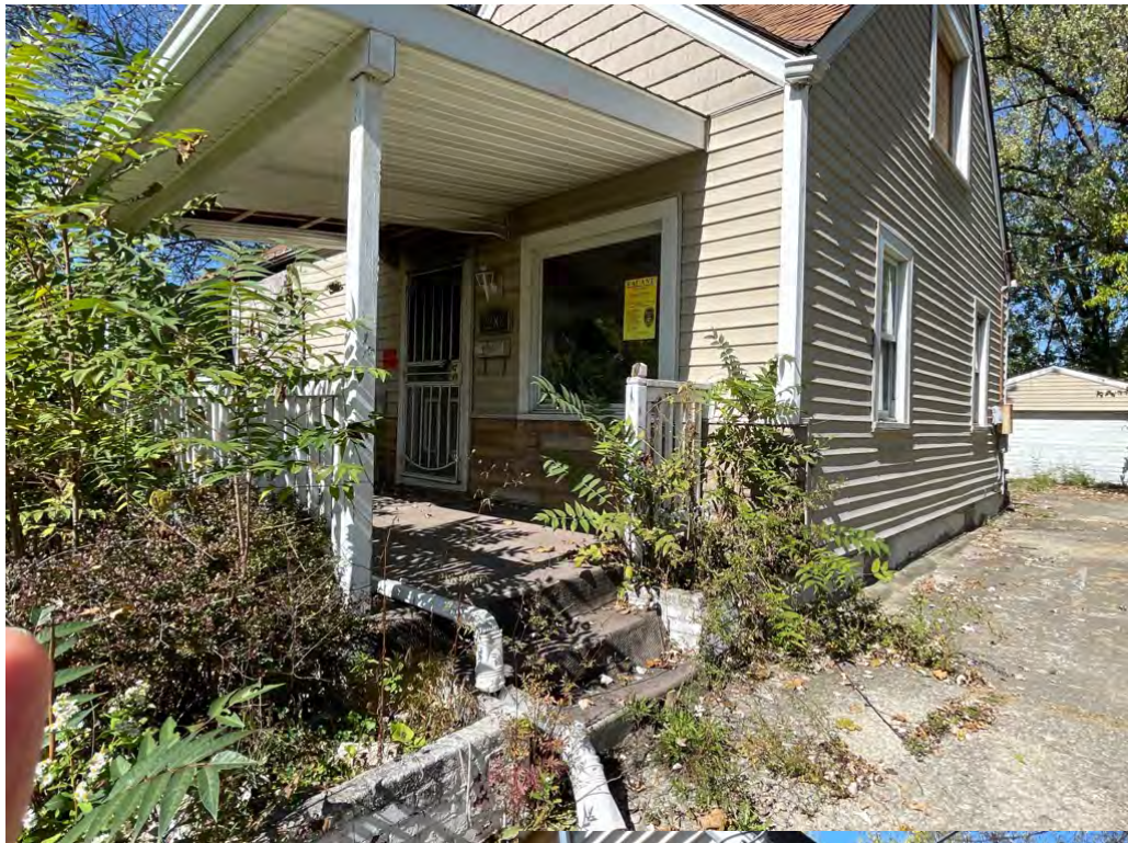
Vacant structure not boarded to code. Bare, exposed wood surfaces present on exterior. Damaged and/or missing sections of siding. Rain carriers full of debris. Missing downspout. High grass/weeds.
