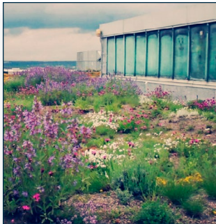
An award winning green development, the Lazarus Government Center was one of the first buildings in Central Ohio to include a green roof.
