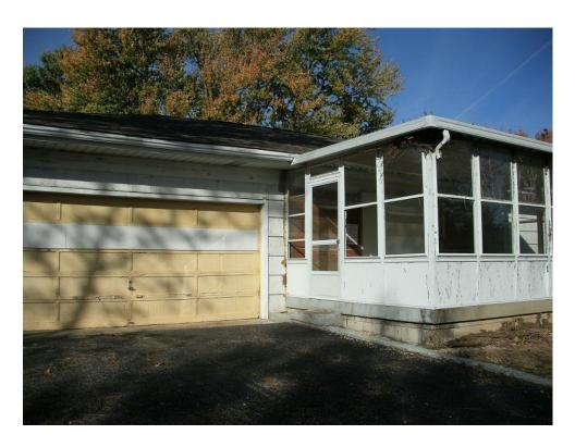
This view shows the garage and sun porch area and the associated continued poor condition of the shingle siding along with peeling paint.
