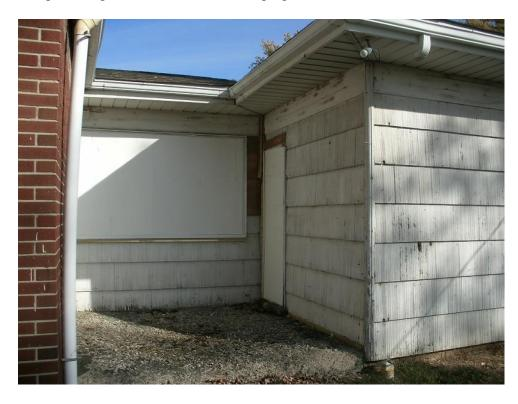
This view just to the right of the Slide C image shows the poor condition of the paint along with damaged and missing shingles from the siding.
