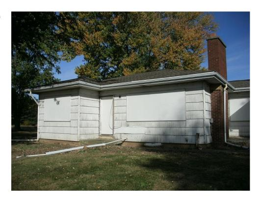
This view of the front entry way of the structures shows the worn condition of the shingle siding and front door trim hanging loose.
