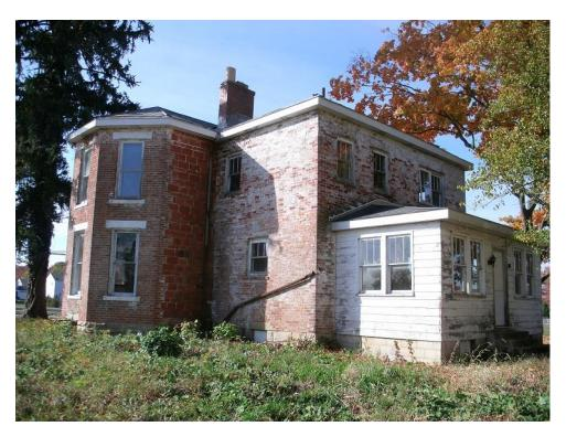
This view again shows the rear of the structure. Note the loose, hanging downspout and overgrown landscaping.
