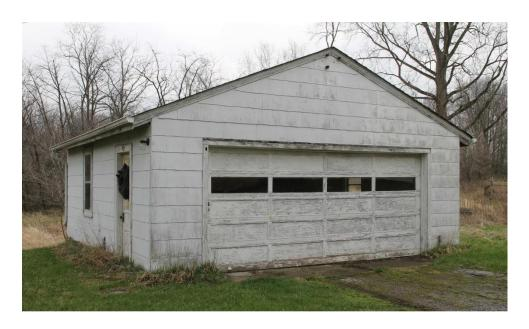
This view shows the general poor condition of the garage highlighted by the deteriorated paint on the door, the door frame and the siding.
