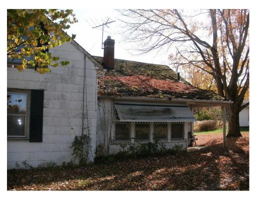
This view shows the poor condition of the siding, roof and window awning. Also note the overgrown vegetation.
