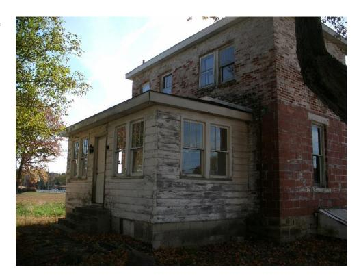
This view shows the general poor condition of the rear of the structure. Note the poor condition of the paint and broken light fixture to the right of the door.
