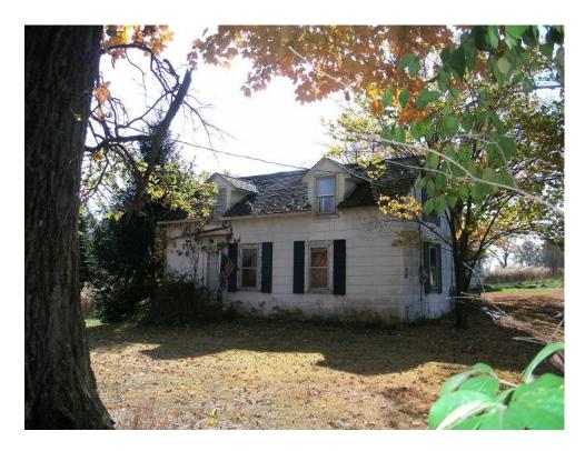
This view of the front of the structure shows mildewed siding along the lower front right corner continuing to the side. Also note the overgrown vegetation at the front door.
