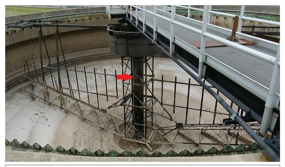
Shown above is a Gravity Thickener at Jackson Pike which is used to remove water from primary waste before the waste goes to the storage tanks. The Center Pier that the red arrow is pointing to conveys the primary waste into the tank. The Center Pier is also the structural support for the gear box, the scrapers, and the walkway.
